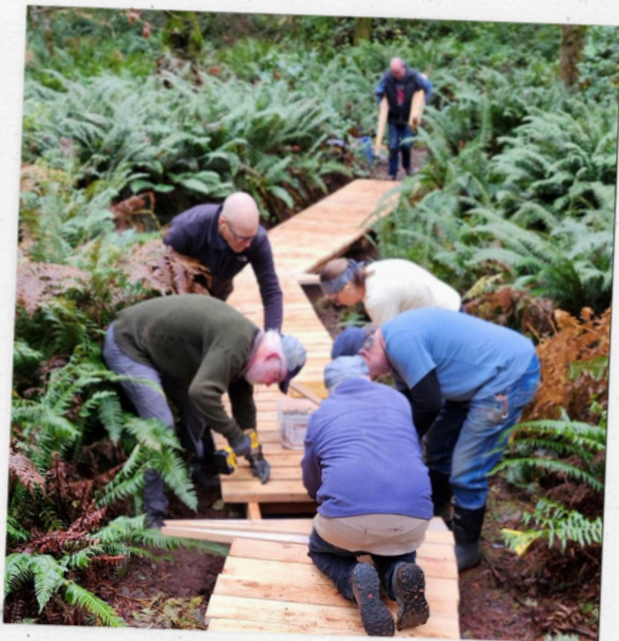
In Elder Cedar (S'ul-hween X'pey) Nature Reserve we created 22m of new boardwalk to protect from foot traffic.
