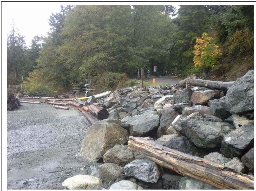
Foreshore Modification Structure: Hard Armouring Riprap ("stacked boulders) intruding into the foreshore. Photo: RC de Graaf
