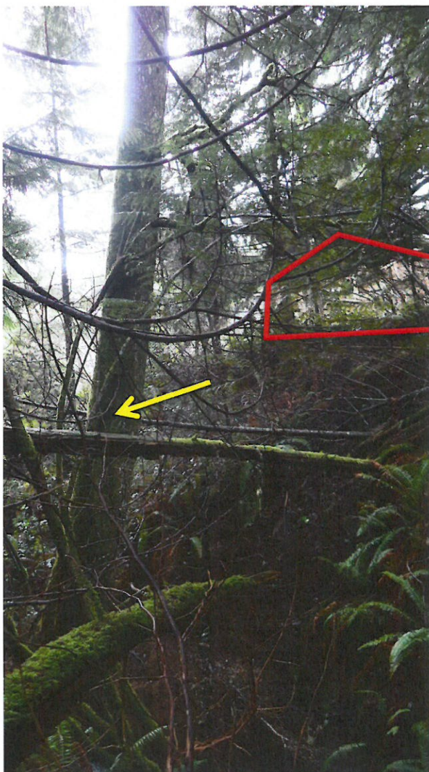
Figure 18: Large western hemlock tree (yellow arrow) that has been undermined by Cicero Slough Creek (yellow arrow) leans towards the existing house (red polygon).
