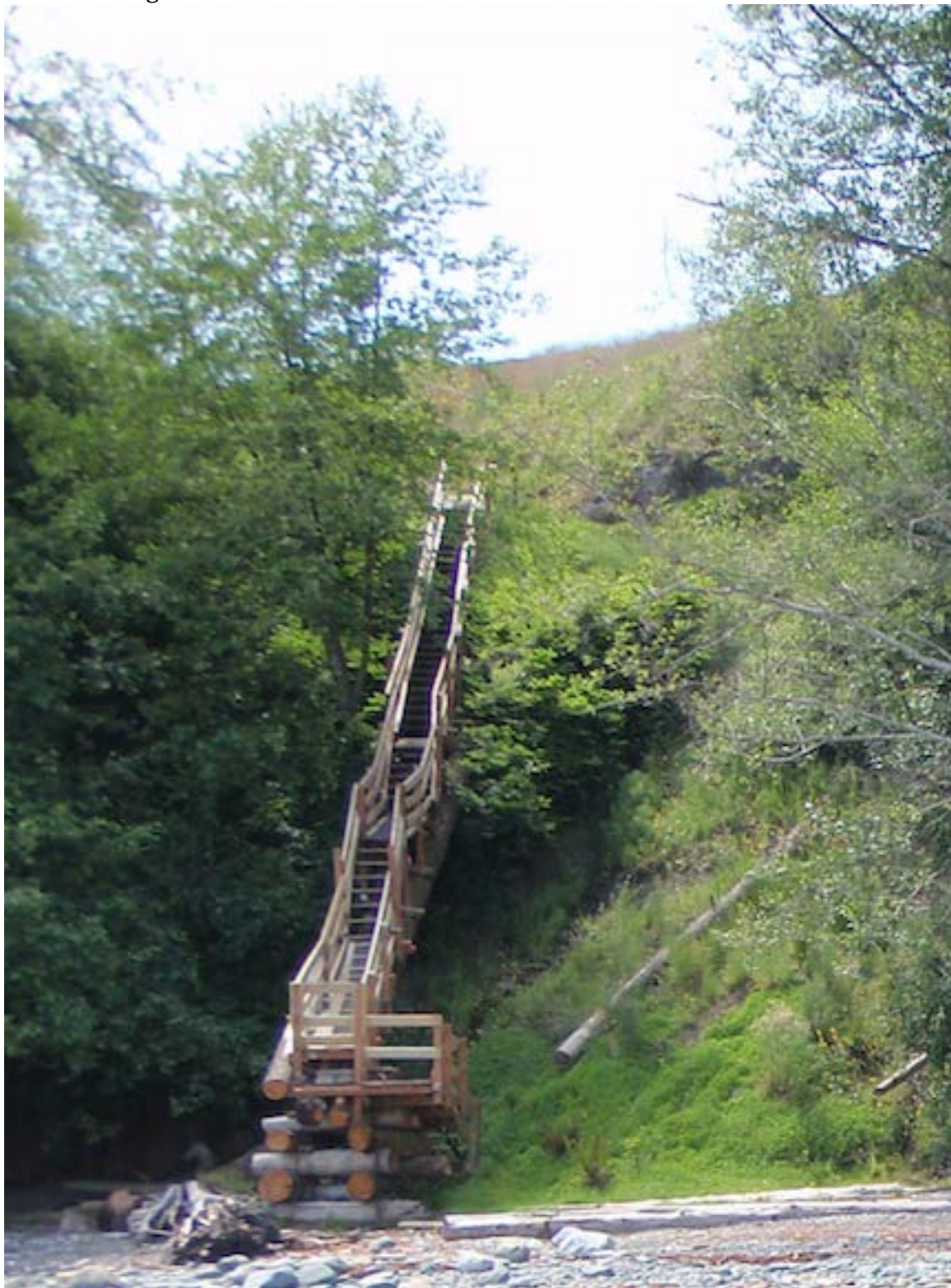
After Planting Remediation
