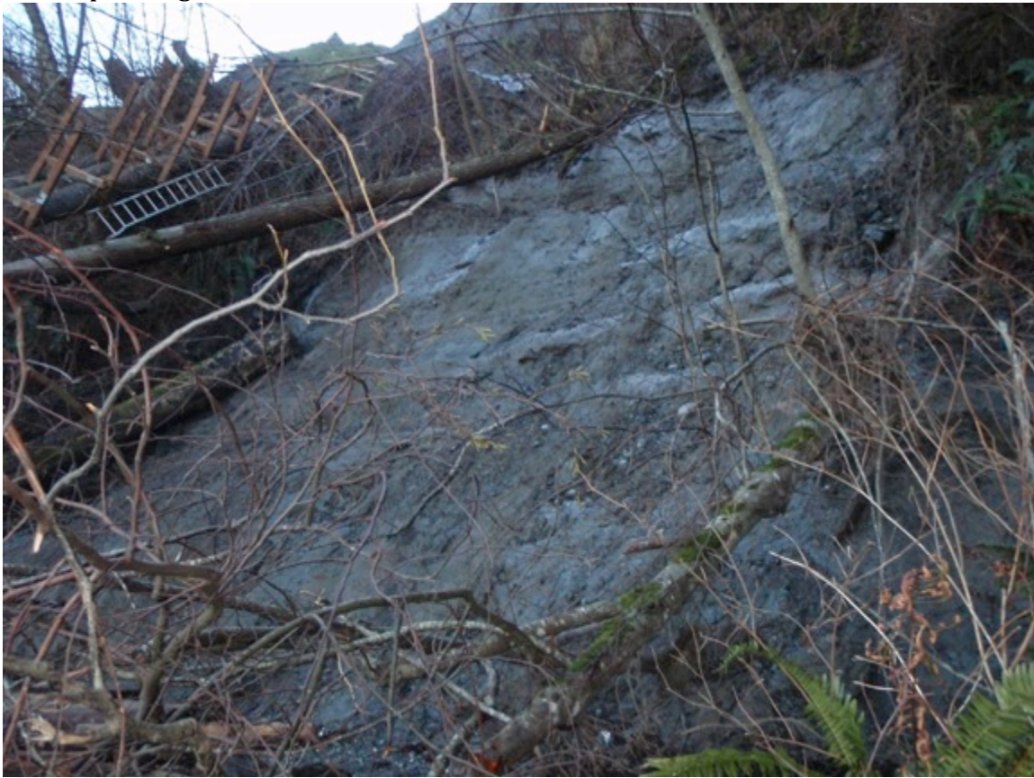
Before planting remediation below stairs
