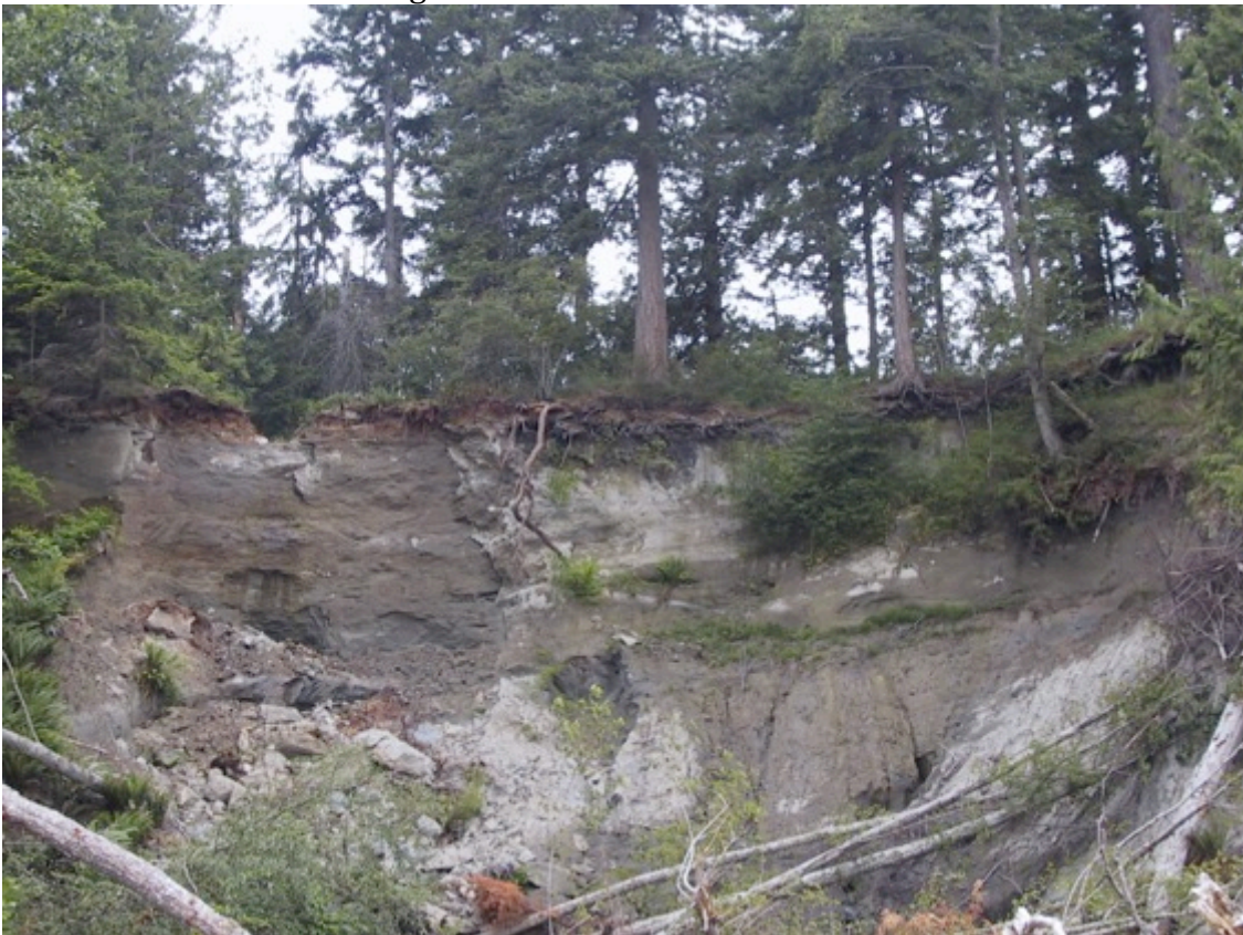
Remaining undermined hazard trees from 2004
