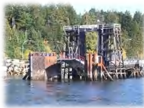
Denman Island Ferry Dock
