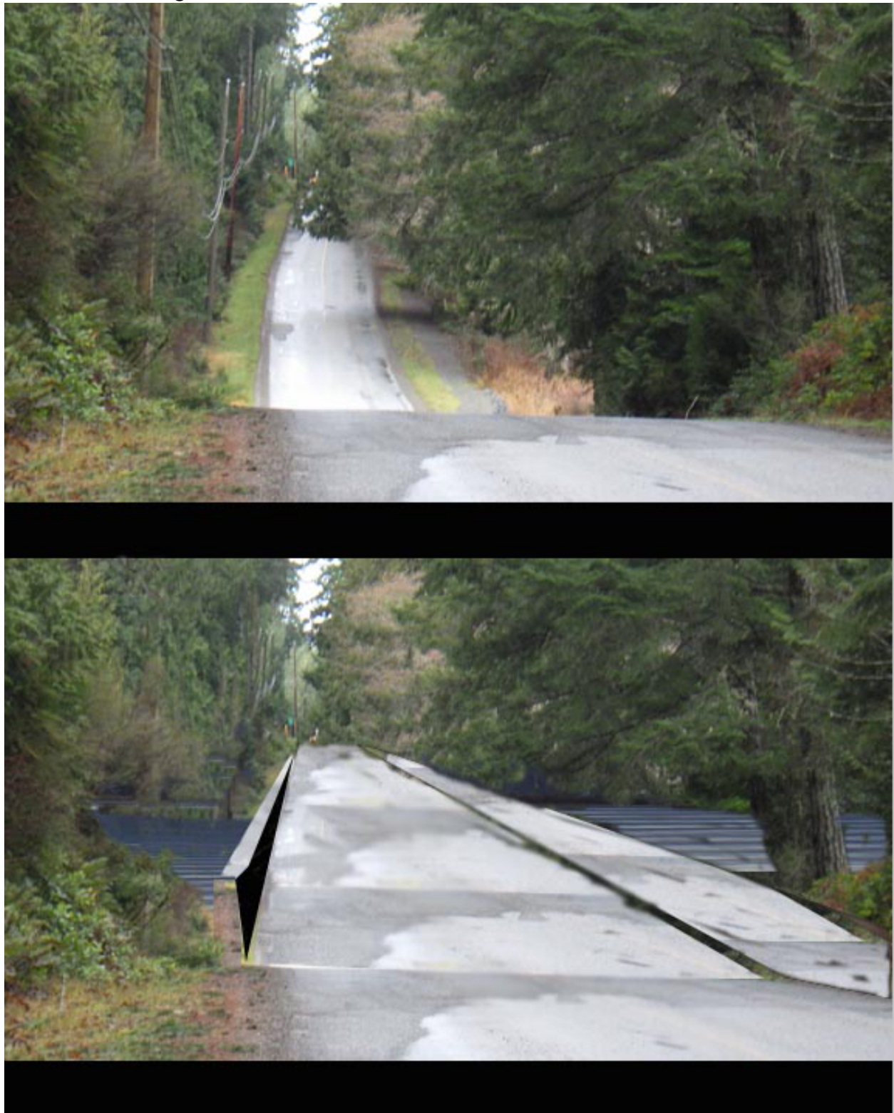
Photo of existing Denman Road and new road elevation:
