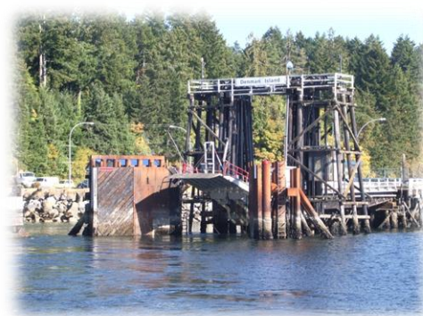
Denman Island Ferry Dock
