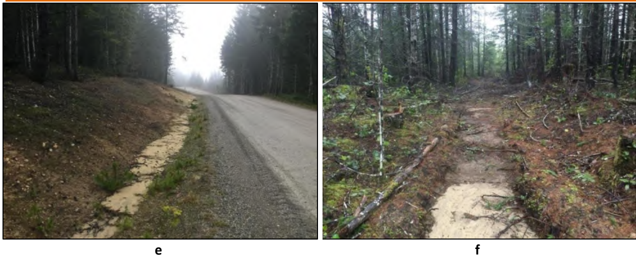
Figure 8, representative photos of Ditches 4 (a, b), 5 (c, d) and 6 (e, f). Photos on left are upslope within the ditch and photos on the right are downslope towards where they infiltrate the ground.
