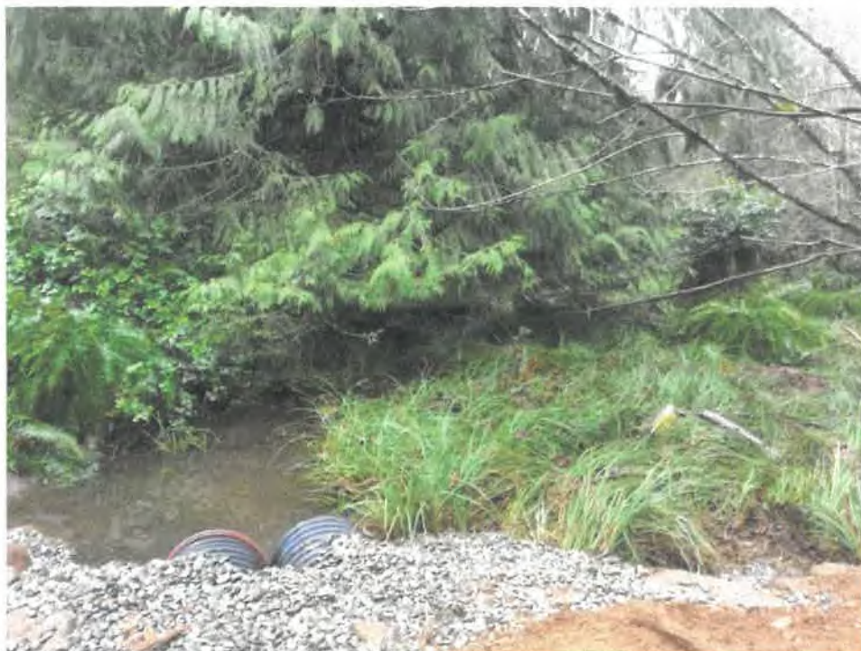
Photo 2. Downstream view of the outlets of the two newly installed culverts in Valens' Brook. Note channel width at left is 14 approx. 1.5 m while floodplain at right is 5 m wide.
