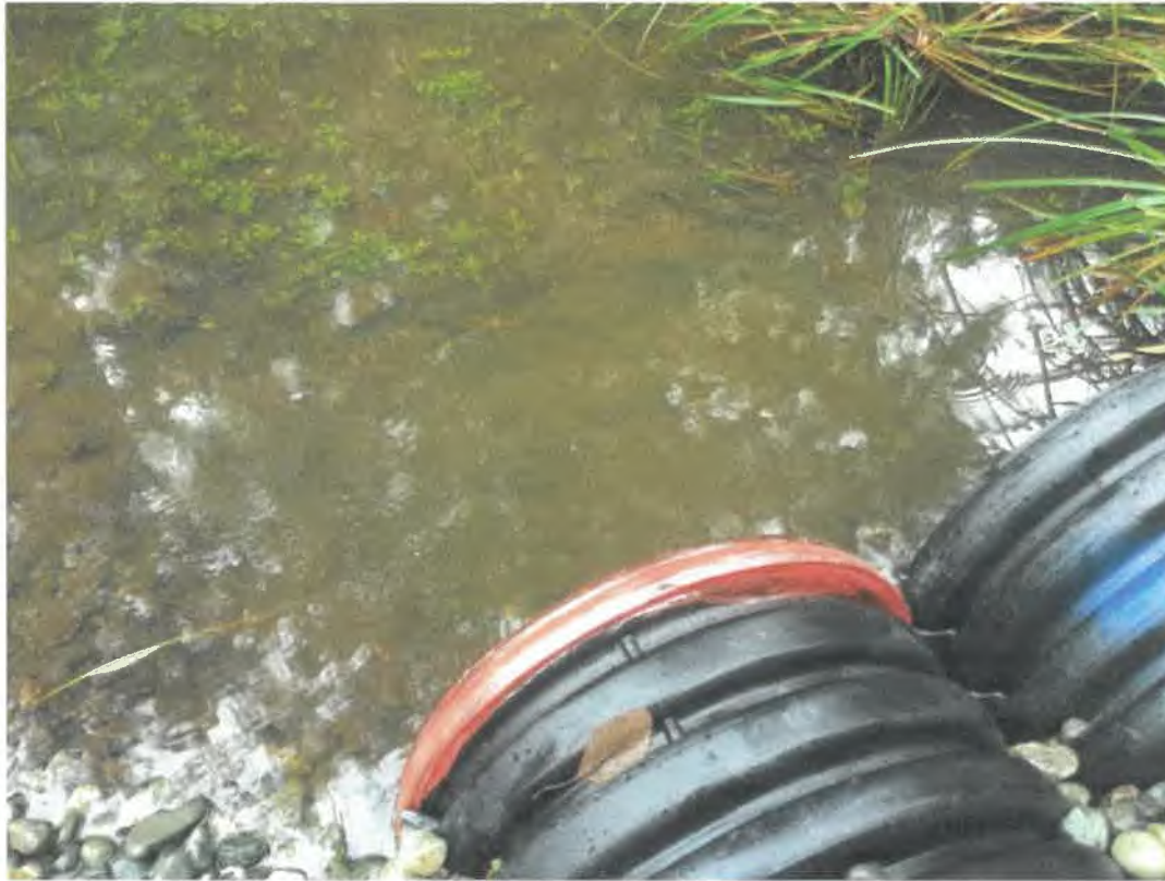
Photo 5: The downstream end of the two culverts with the outlet pool invert visible and minor scour to be substrates resulting from concentrated flows that will be diffused by the addition of a third culvert.
