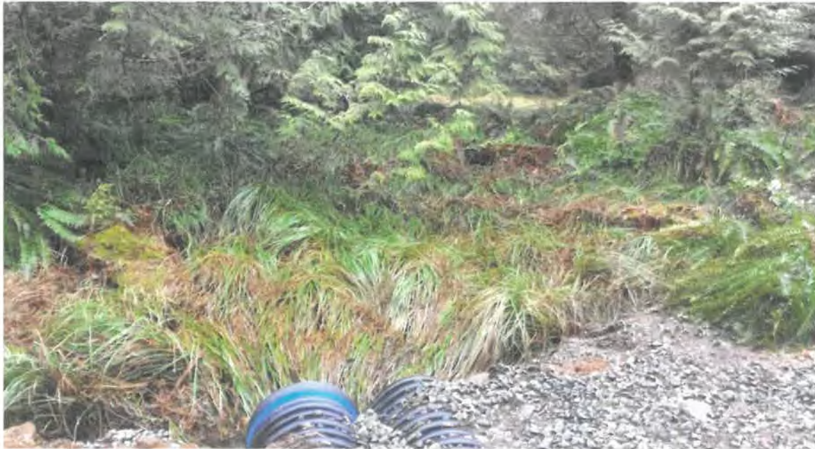
Photo 8: The upstream end of the culverts installed in Valens' Brook. Note the lack of a clearly defined channel free of vegetation (in contrast to Photo 2 above of the outflow). Both up and downstream sides of the crossing will be upgraded by installing non-woven geotextile over its banks and covered with larger diameter rock to avoid erosion of fine materials.
