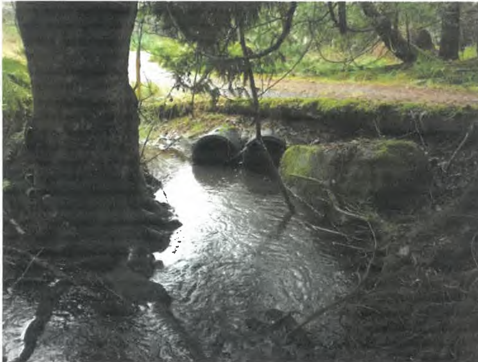
Photo 6: Twin 0.45 m diameter culverts installed under Tristone Road approximately 140 m downstream of the crossing on the subject property.
