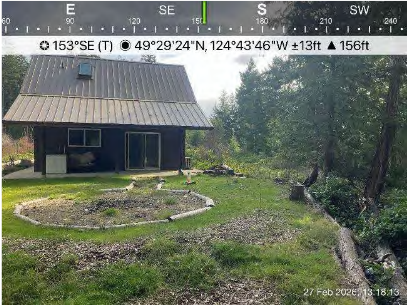
PHOTO 4. VIEW LOOKING AT THE REAR OF THE ACCESSORY BUILDING AT UNPERMITTED FILL IN AN APPROXIMATE AREA OF 10M BY 10 M ALONG THE EDGE OF THE STEEP SLOPE AND WITHIN DPA 2.
