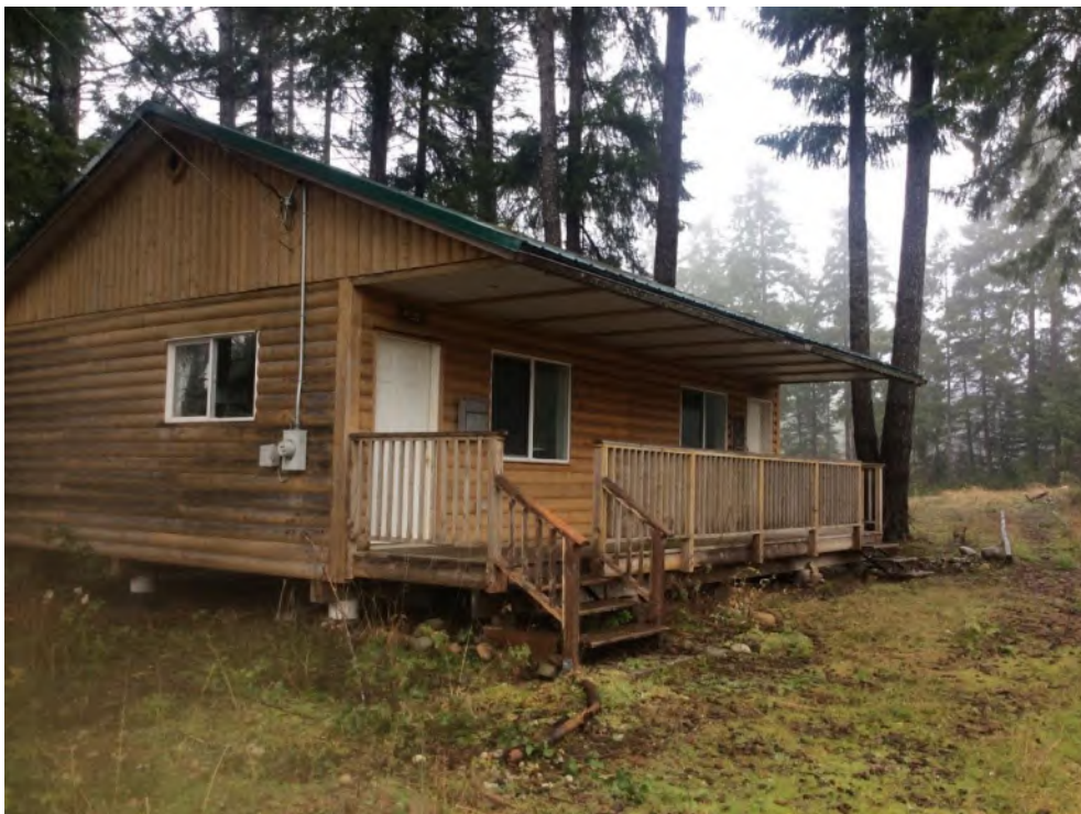
Photo 11: Existing temporary structure to be removed before development.
