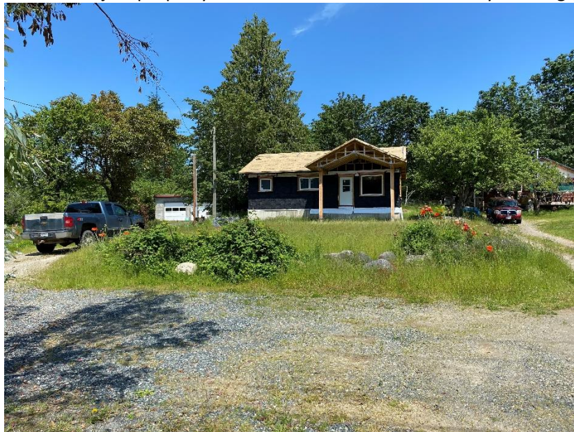
View facing the subject property from Denman Road.
