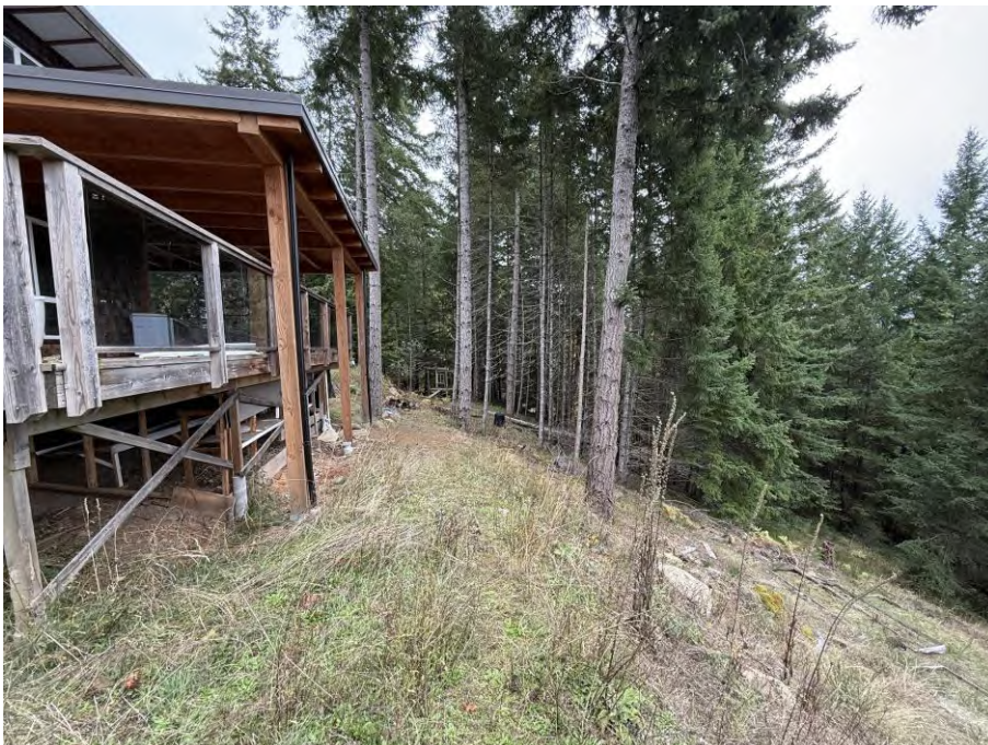
PHOTO 2. VIEW SOUTHWEST OF THE HOUSE THAT WAS CONSTRUCTED ON THE SUBJECT PROPERTY IN 2016, SHOWING THE TRANSITION TO STEEP SLOPE HABITAT, WHERE VEGETATION CLEARING OCCURRED BETWEEN 2016 AND 2018.
