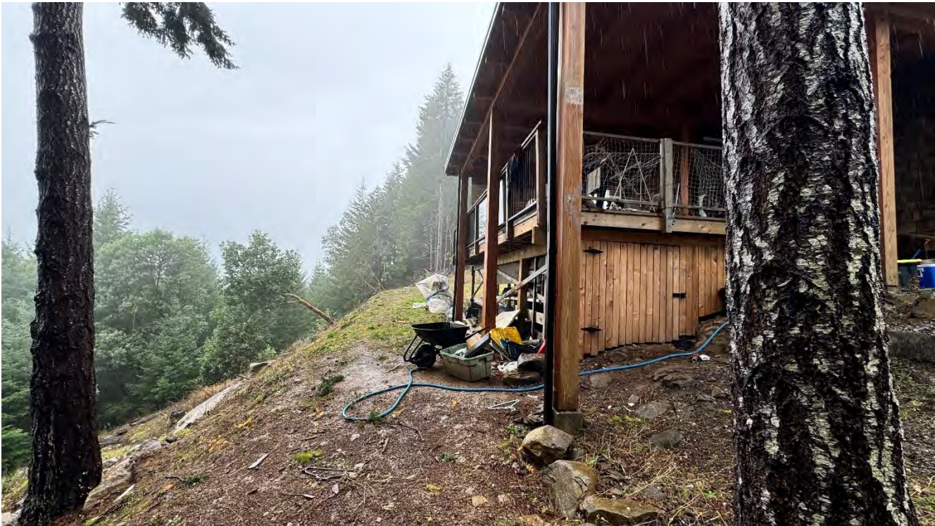
Photo 2.2.1 – Slope conditions at crest of slope, looking approximately northwest.
