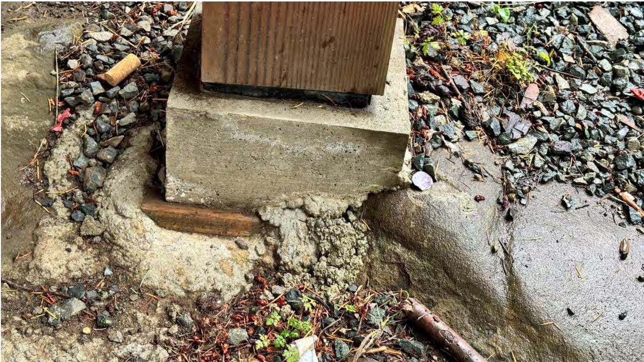
Photo 2.4.2 – Pad footing on southern side of SFR on sandstone bedrock.
