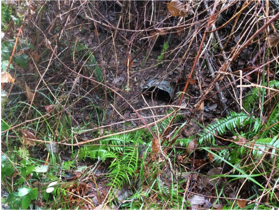
Photo 10: Culvert draining to the wetland from the municipal works yard to the north of the subject property.
