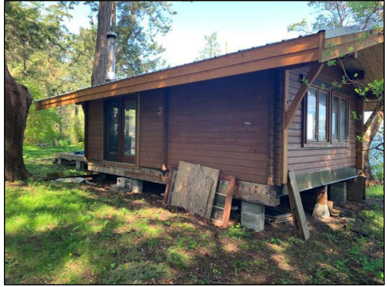
Photo 5. Showing the back of the cabin facing northwest. The timber-frame cabin is supported by concrete piers.
