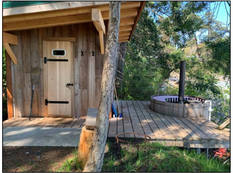
Photo 13. A small deck with wood-fired hot tub and sauna is located to the northwest of the cabin. The structure was constructed 3 years ago at the top of bank of the foreshore slope that leads down to the beach.
