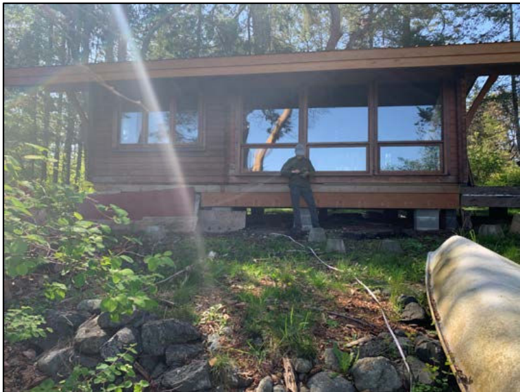
Photo 6. Showing the north side of the existing cabin that faces the ocean. The deck has been removed.
