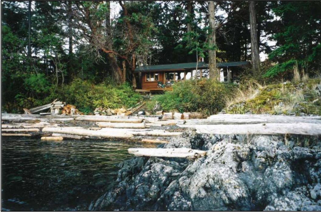
Photo 1. The subject property on Mistaken Island, BC showing the small cabin that was built in 1957 7.9m from the present natural boundary of the eastern shoreline within the southern portion of the island.
