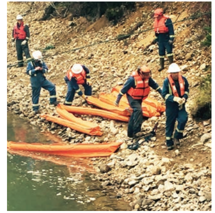
Emergency and spill response booms specifically selected for water-based spill containment and recovery
