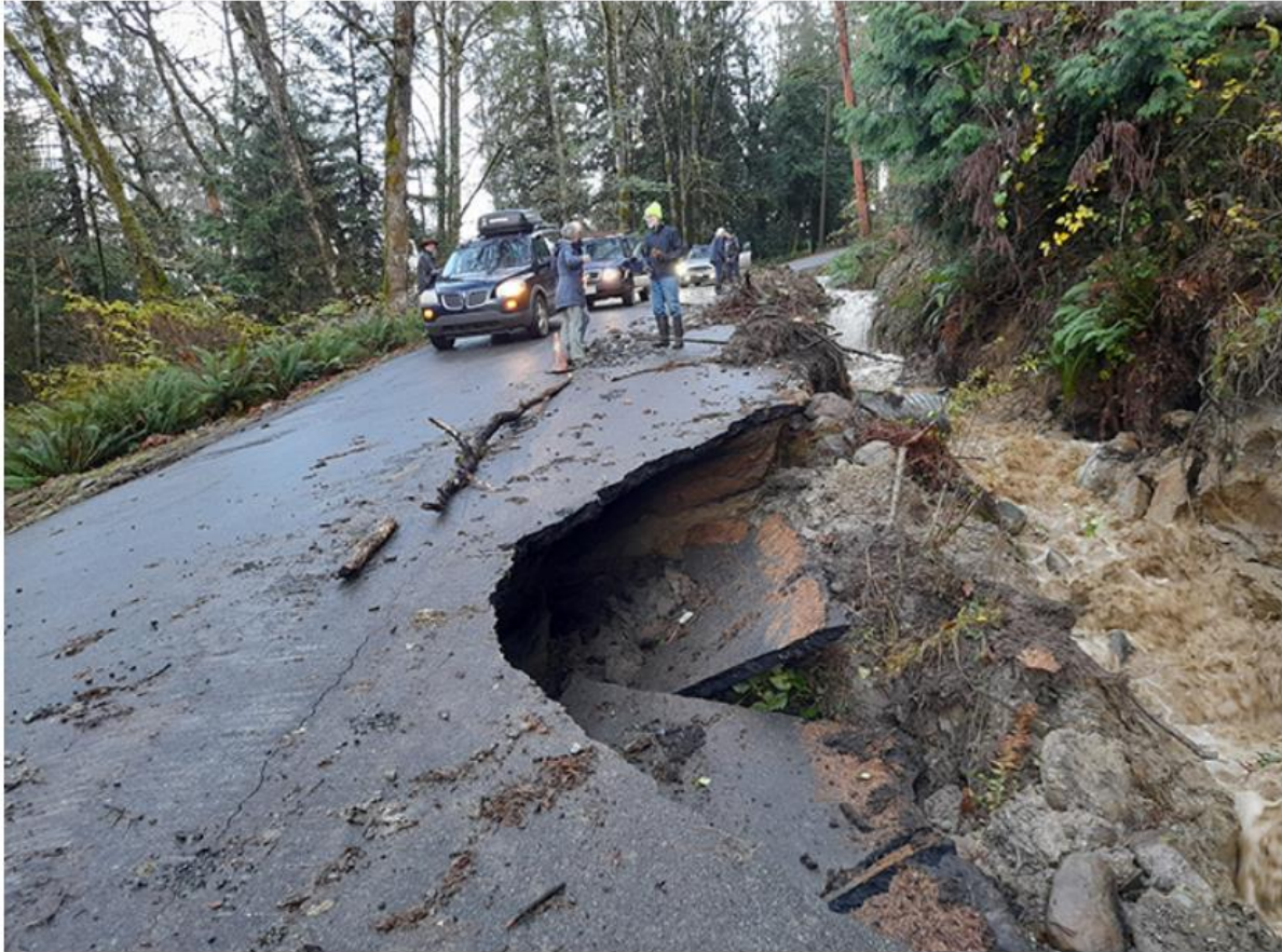
Damage in the form of a washout and erosion caused by heavy rains at the junction of Roland Road and Isabella Point Road at 3 p.m. on Nov. 15.
