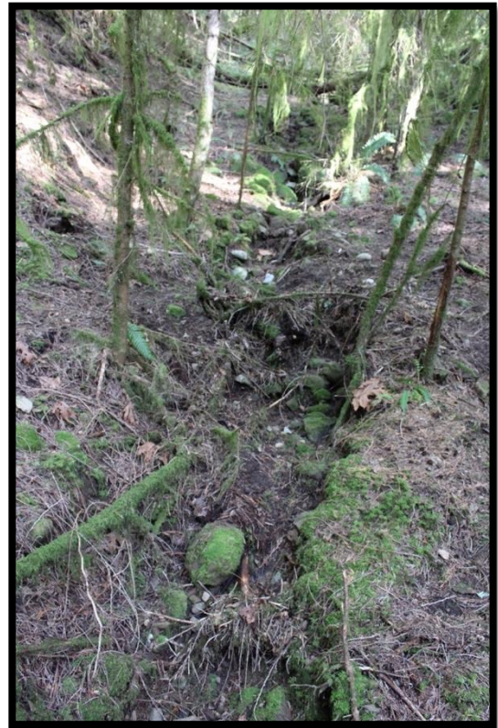
Photo 11. Erosion caused by seasonal creek flowing along old road.
