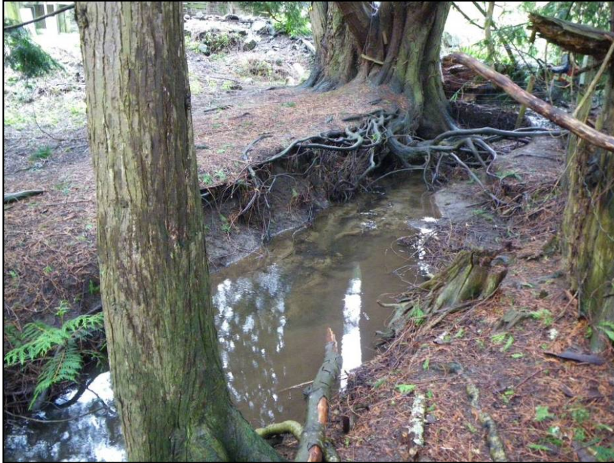
Typical example of unstable banks found in the upper reaches of the Lyall Creek tributary drainage. Note sparse nature of riparian vegetation, which has led to a decrease in the function of bank stability.
