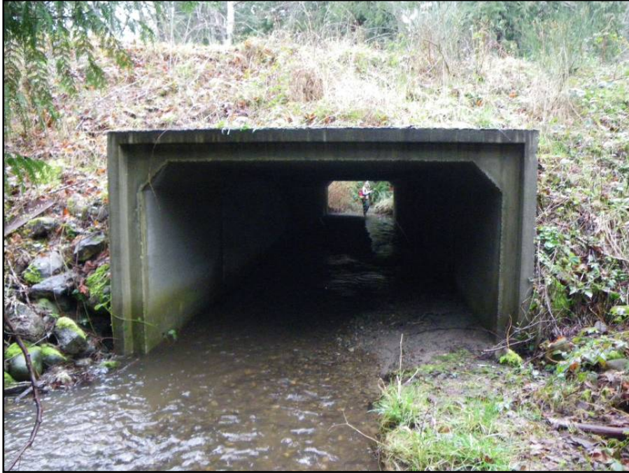
Looking downstream (northwest) through the open-bottomed box culvert structure located on the first road crossing above tidewater.
