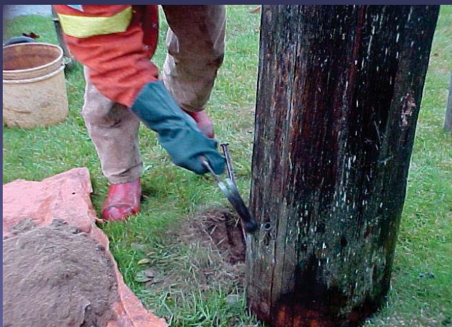
Installing Plugs
