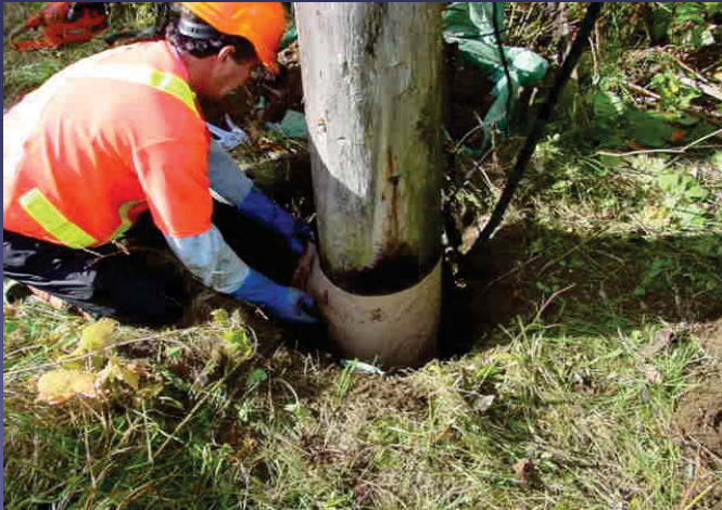
Installing a full bandage
