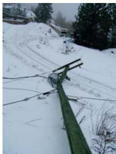
Public Safety Hazard
