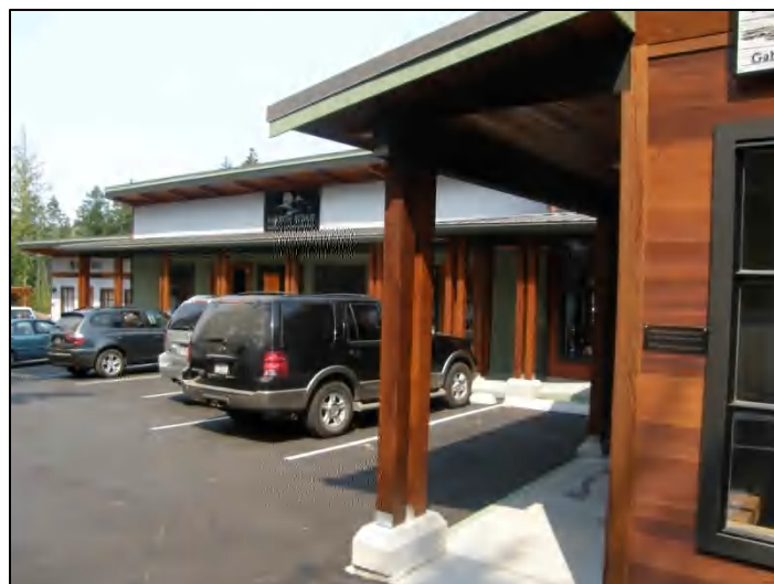
Figure 5: Madrona Marketplace Phase 1 – East Building
