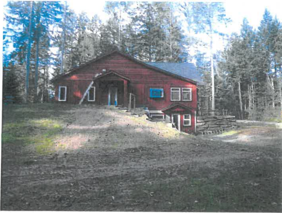
Looking west through the SPEA towards the recently-constructed residence.
