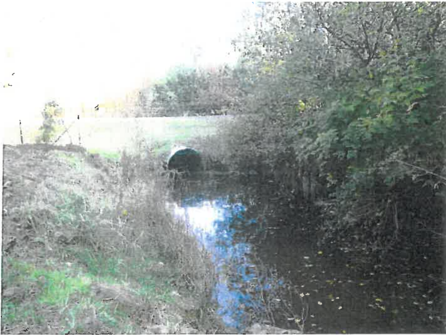
Looking upstream (North) along Goodhue Creek where it enters the subject property via a culvert under Wildwood Crescent.
