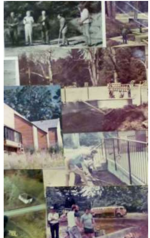
Figure 63: Construction photos of the current Hall
