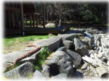
Photo 4. Riprap rock wall built on backshore between the deck and beach.
