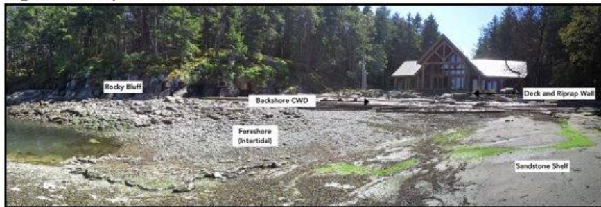
Figure 1. Subject house built on beachfront.
