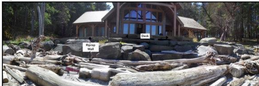
Figure 2. Riprap wall constructed on backshore habitat of shoreline.
