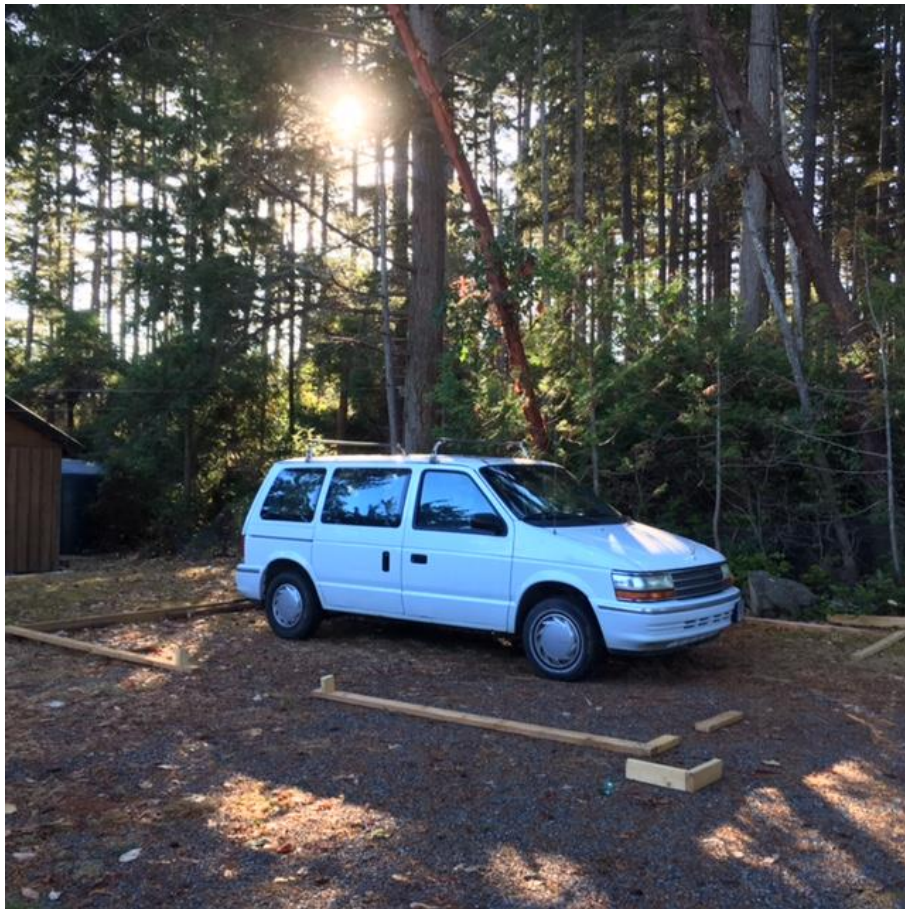
The proposed garage site delineated by boards indicating the location of the footings.
