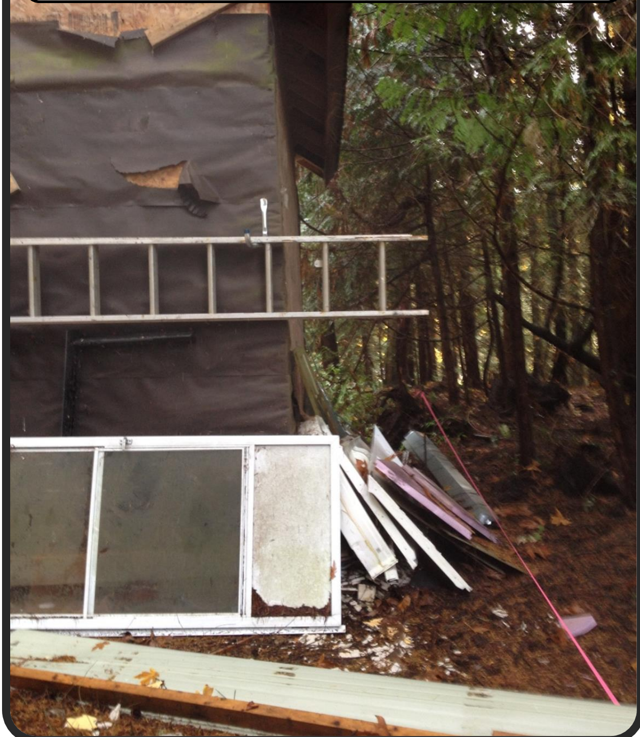
Figure 5: Existing Shed (facing South along western property line)
