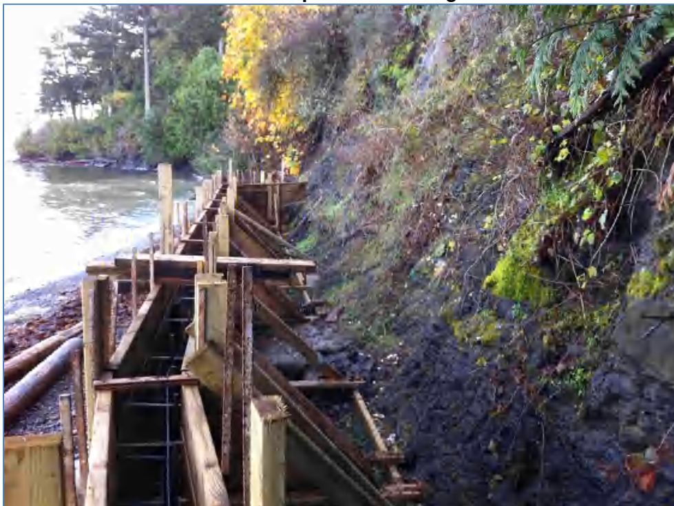
Photo 7: Toe of slope and retaining wall forms
