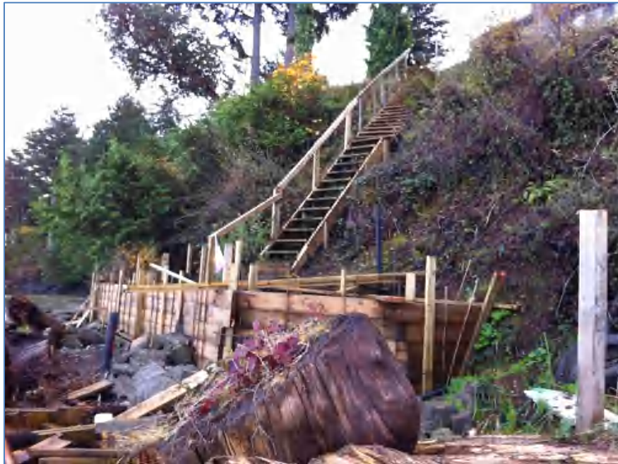
Photo 1: retaining wall formworks, looking Eastward
