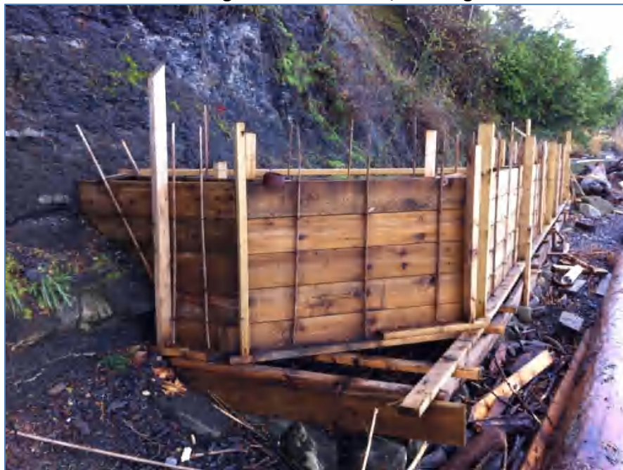
Photo 2: retaining wall formworks, looking Westward
