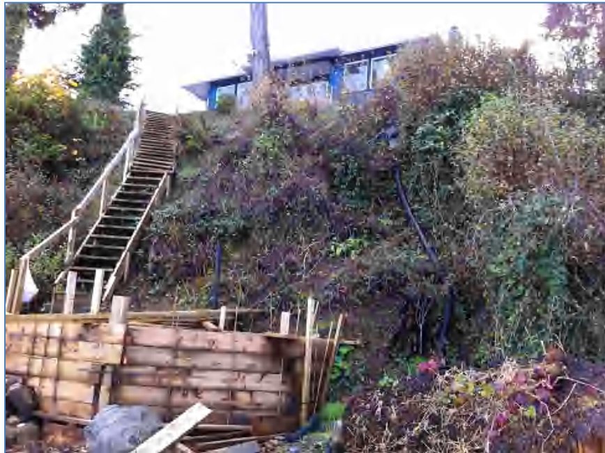
Photo 3: Slope west of stairs
