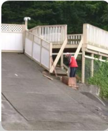
During Construction of Stairs (2012 - 2015)
