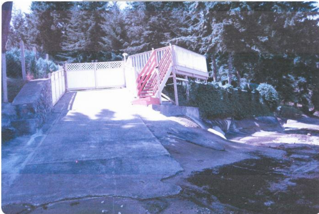
Current view of Boat Ramp and Stairs
