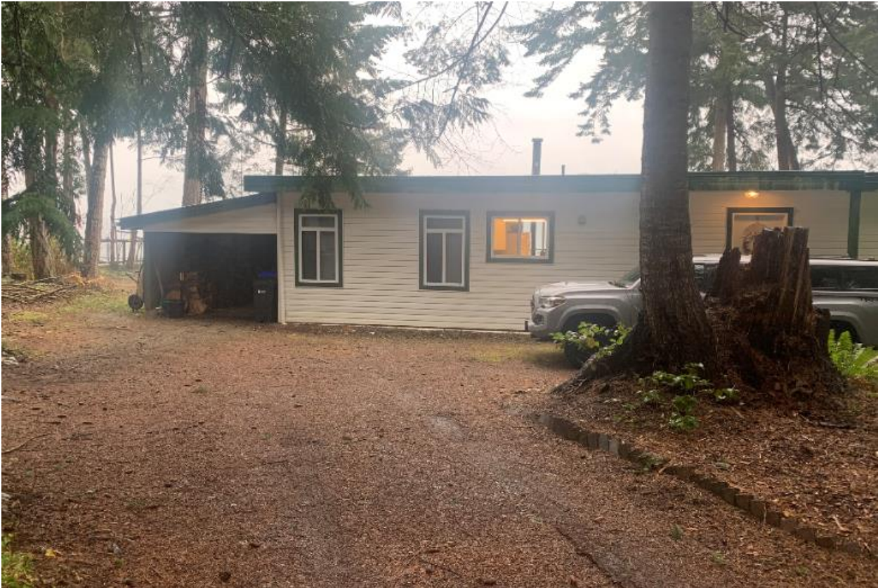
Photo 1: view from the driveway access off Barrett Road.
