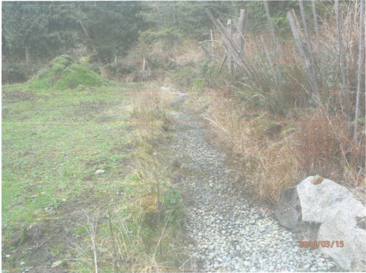
Photo 3. The ditch runs along the west and north sides of the property
