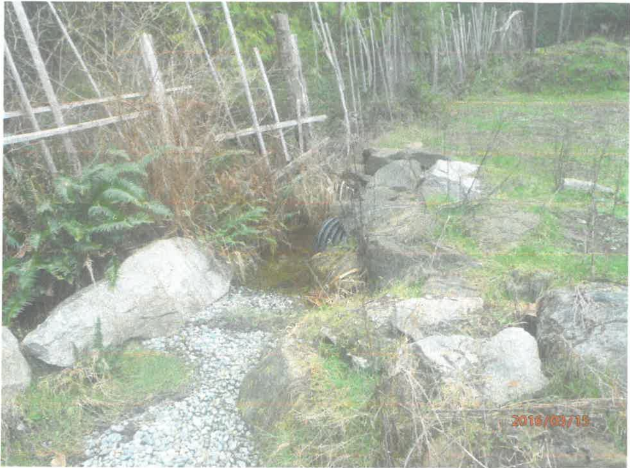
Photo 4. The creek culvert outlet is on the north side of the property
