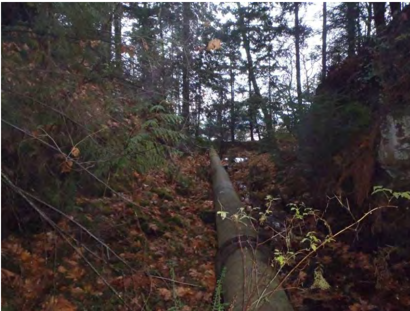
Looking south west from the dam along the outlet pipe. The pipe drops over a steep slope along the slope break in the approximate centre of the photo to the power generating facility.
