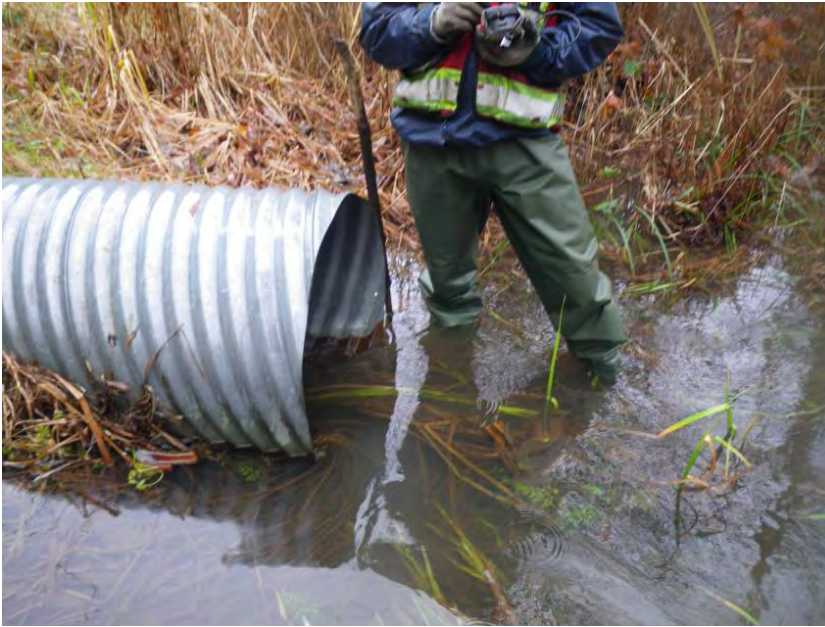
Inflow of culvert upstream of North Road.
