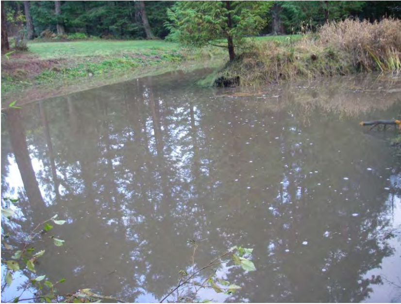
Looking east over an excavated pond that appeared to be constructed by altering the original channel of Dick Brook.
