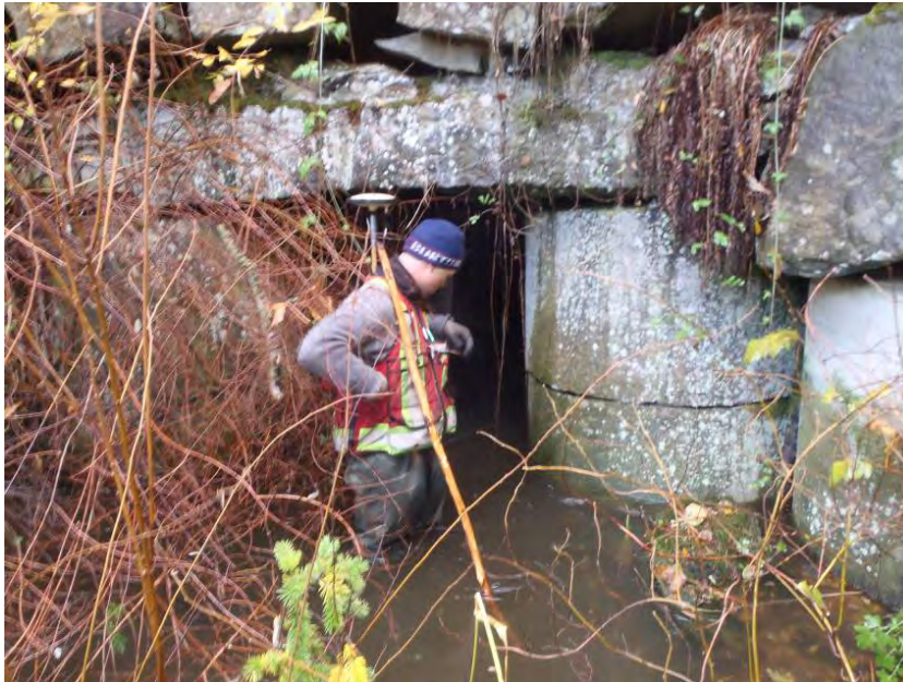
Concrete box-type culvert structure immediately upstream of the golf course on Goodhue Creek.
