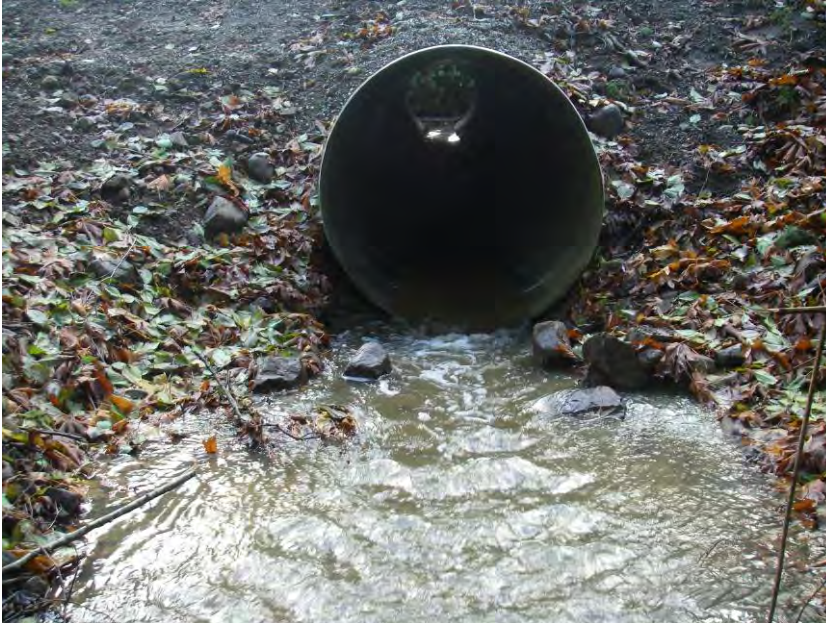
Outflow of the culvert positioned under North Road. It should be noted that this culvert has been recently installed (at the time of writing) as noted by the fresh gravel positioned at both the inlet and outlet of the culvert.
