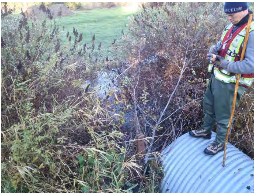
Looking at the inflow of the culvert under South Road on Goodhue Creek.
