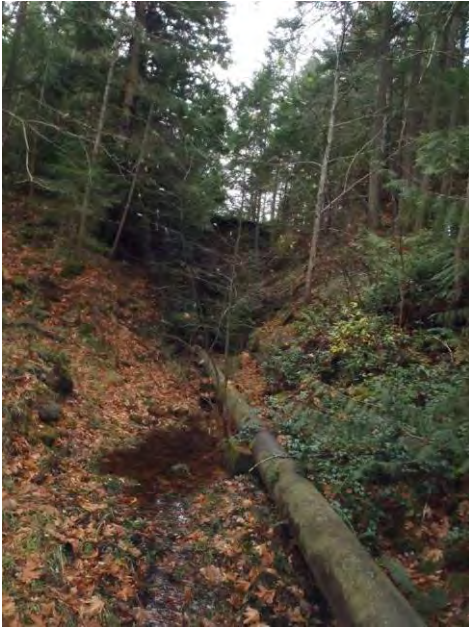
Looking north east towards the dam along the outlet pipe.
