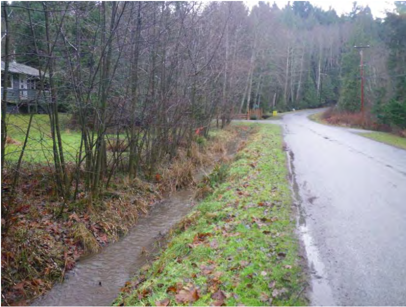
Looking upstream (south west) along Castell Brook where it flows as a roadside ditch adjacent to Bertha Road.
