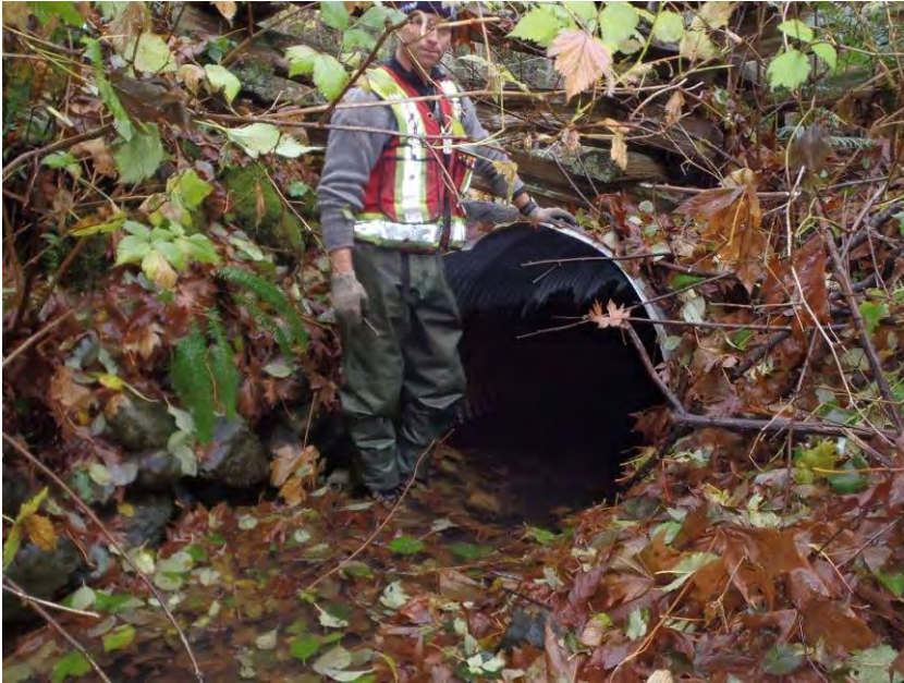
Outflow of the culvert under South Road.
