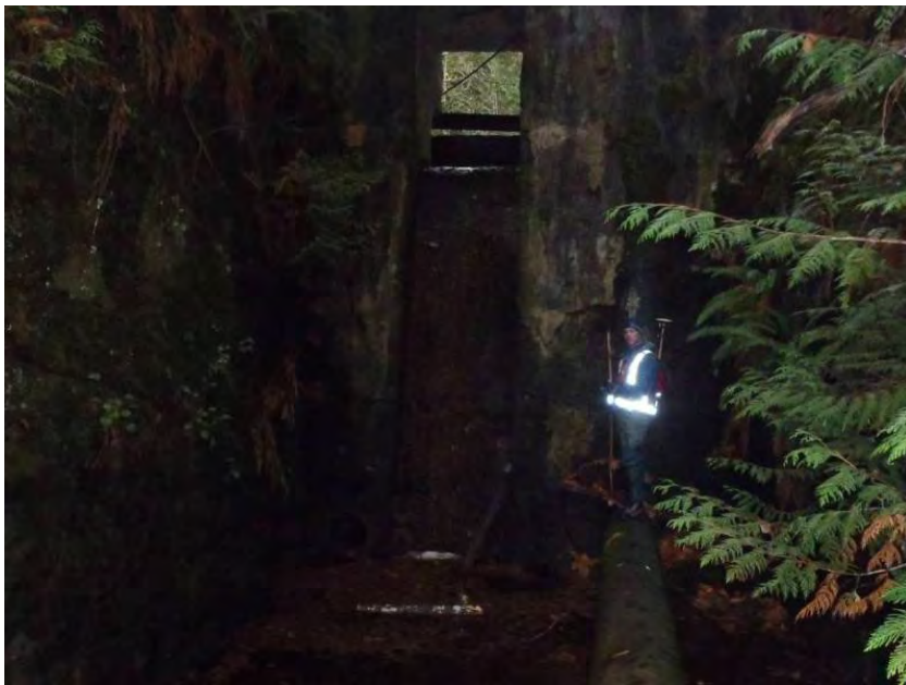
Looking at the downstream side of the dam and weir. Note lack of defined channel below the weir. The pipe takes water from behind the weir for power generation.
