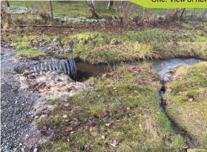
One: View of new culvert in ROW - Eppler Creek
