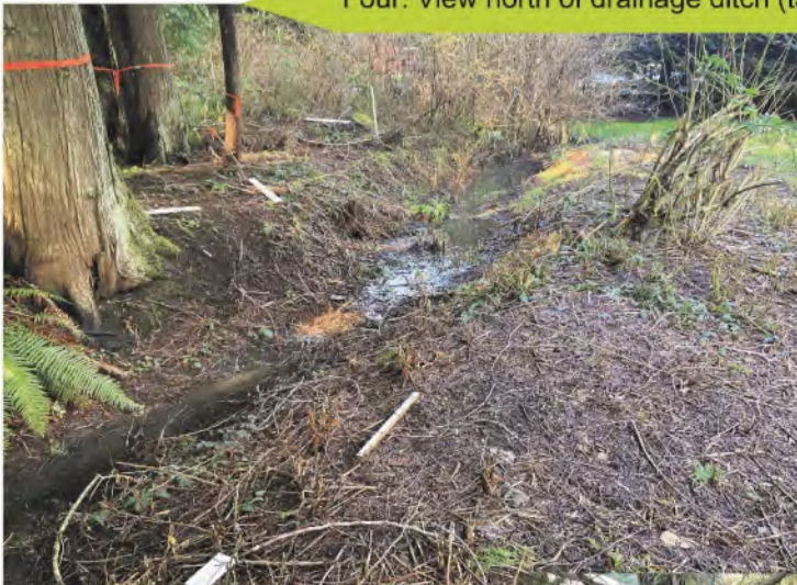
Four: View north of drainage ditch (tagged trees to be removed)
