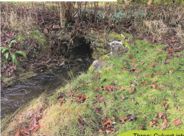
Three: Culvert into property (north east corner)
