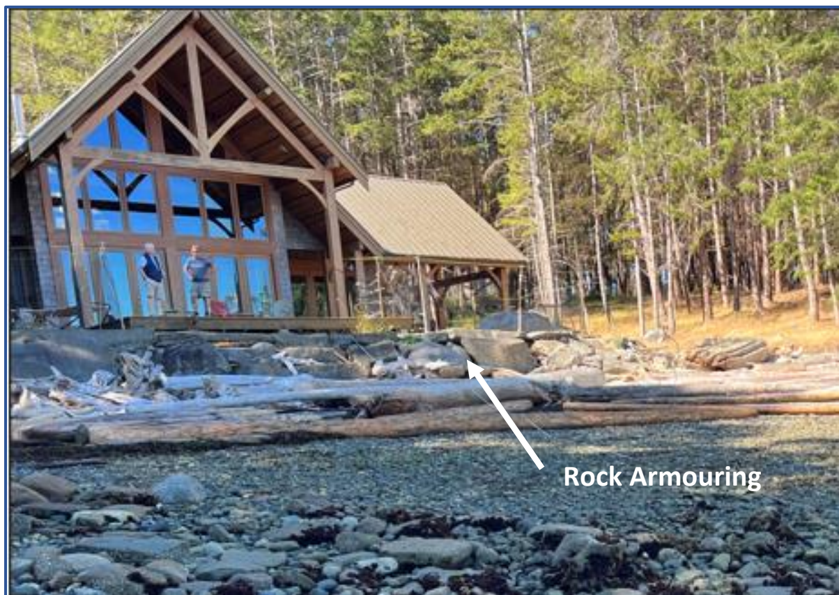
Photo 1 Photograph looking at the rock armouring and upper beach.
