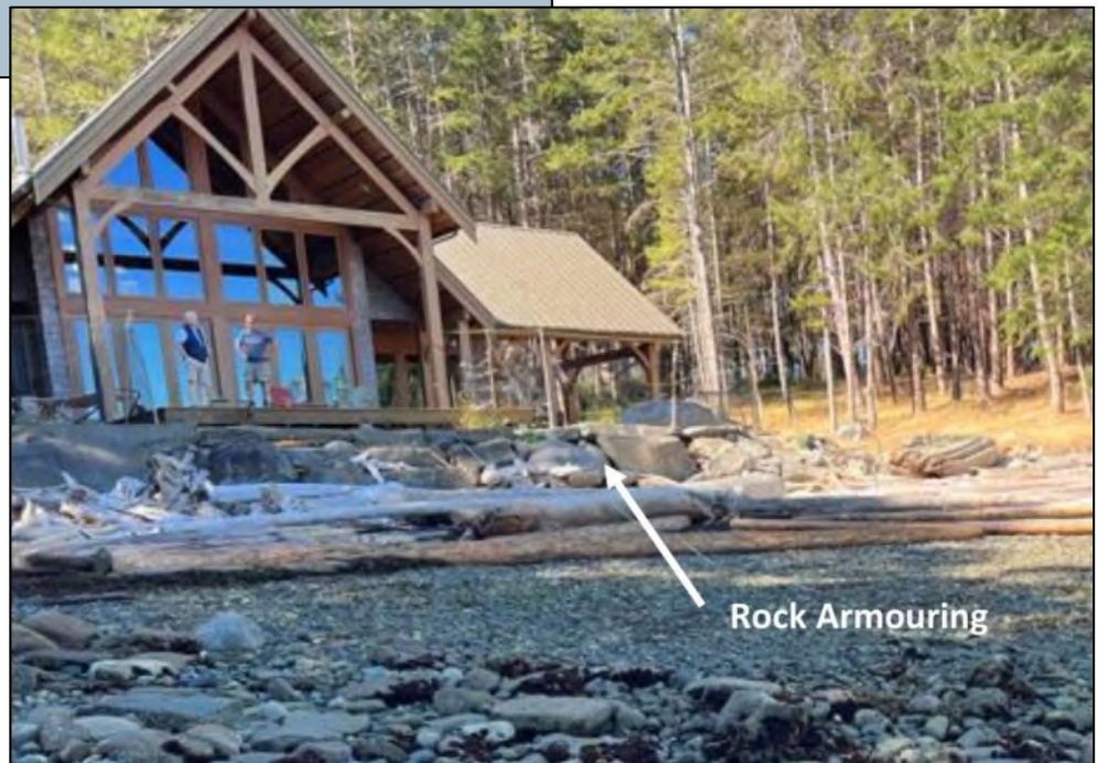
Figure 1 Rock Retaining Wall, also referred to as "Riprap Wall," in front of the house.
