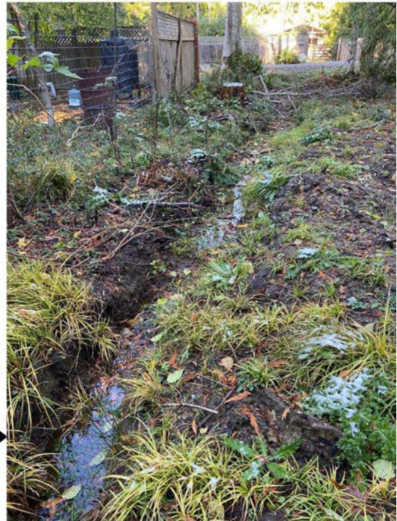
View east of drainage ditch leading to culvert under the driveway
