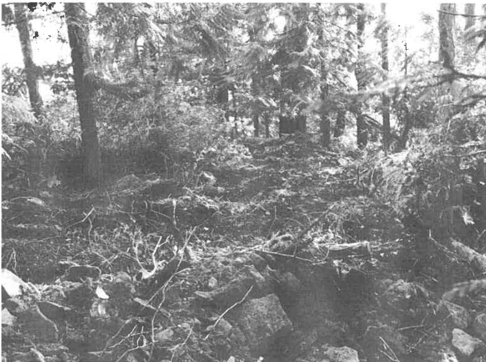
Figure 5: Crest of the Rock Slope Facing East
