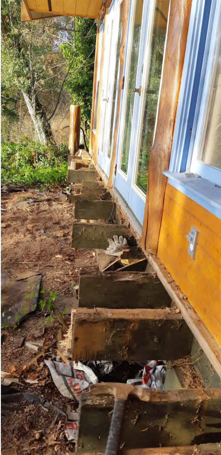
Entrance to Cabana after deck removal
