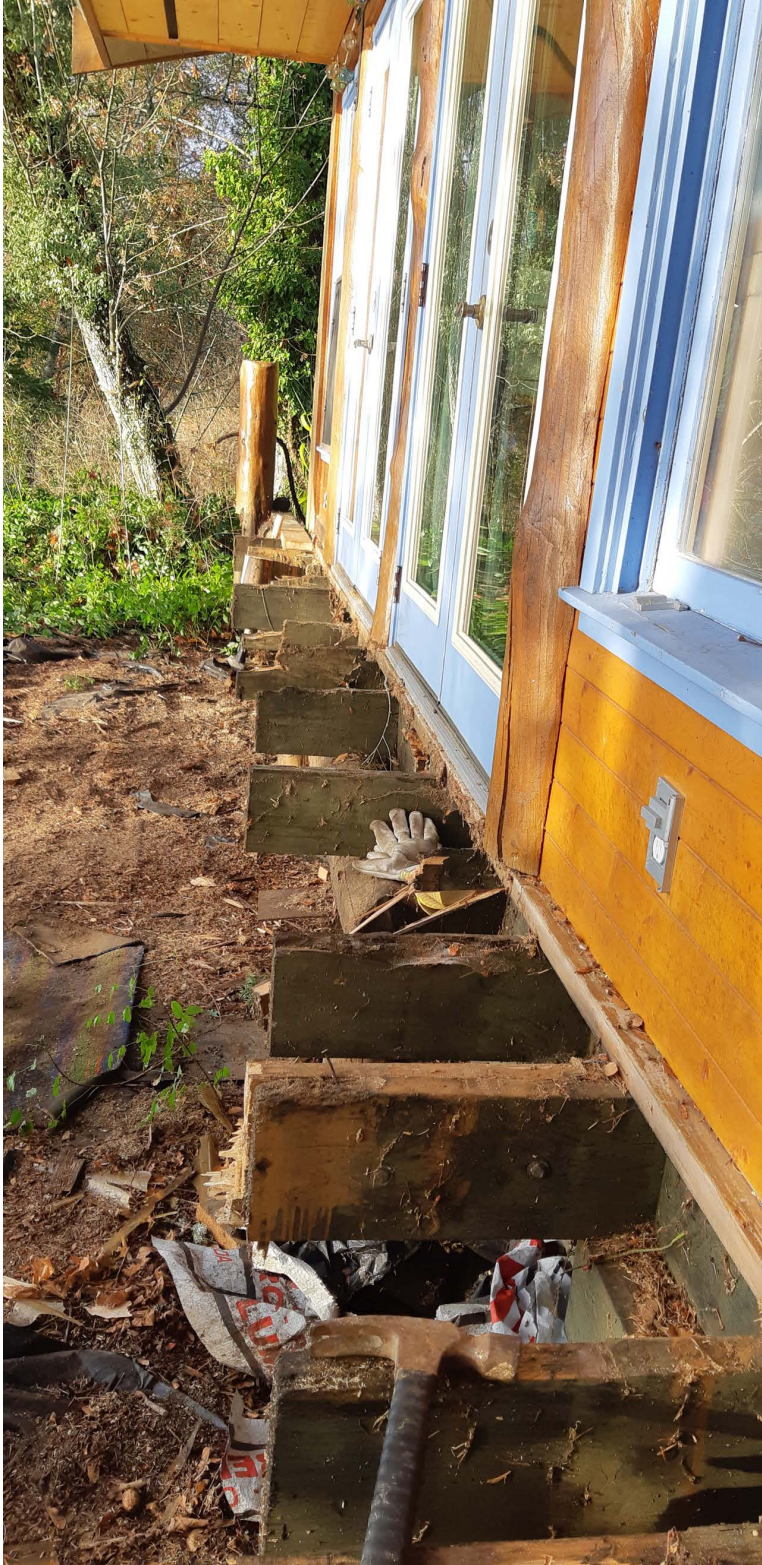
Entrance to Cabana after deck removal
