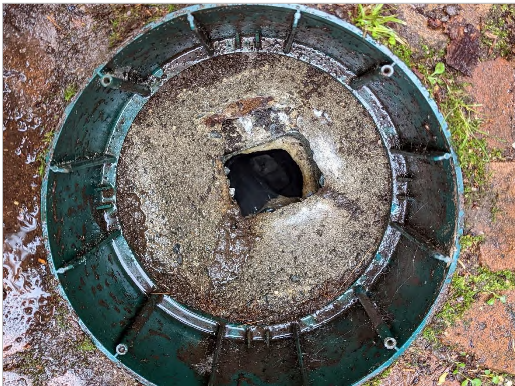
Picture 3: Inlet maintenance hatch
