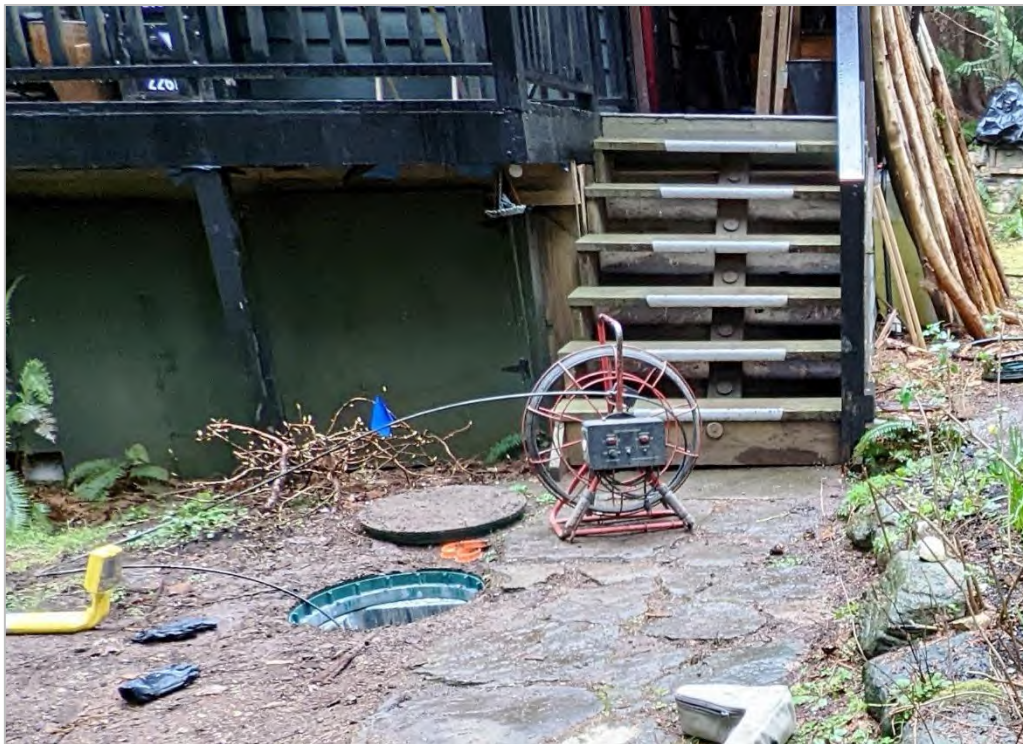
Picture 5: Location of distribution box (d-box)
