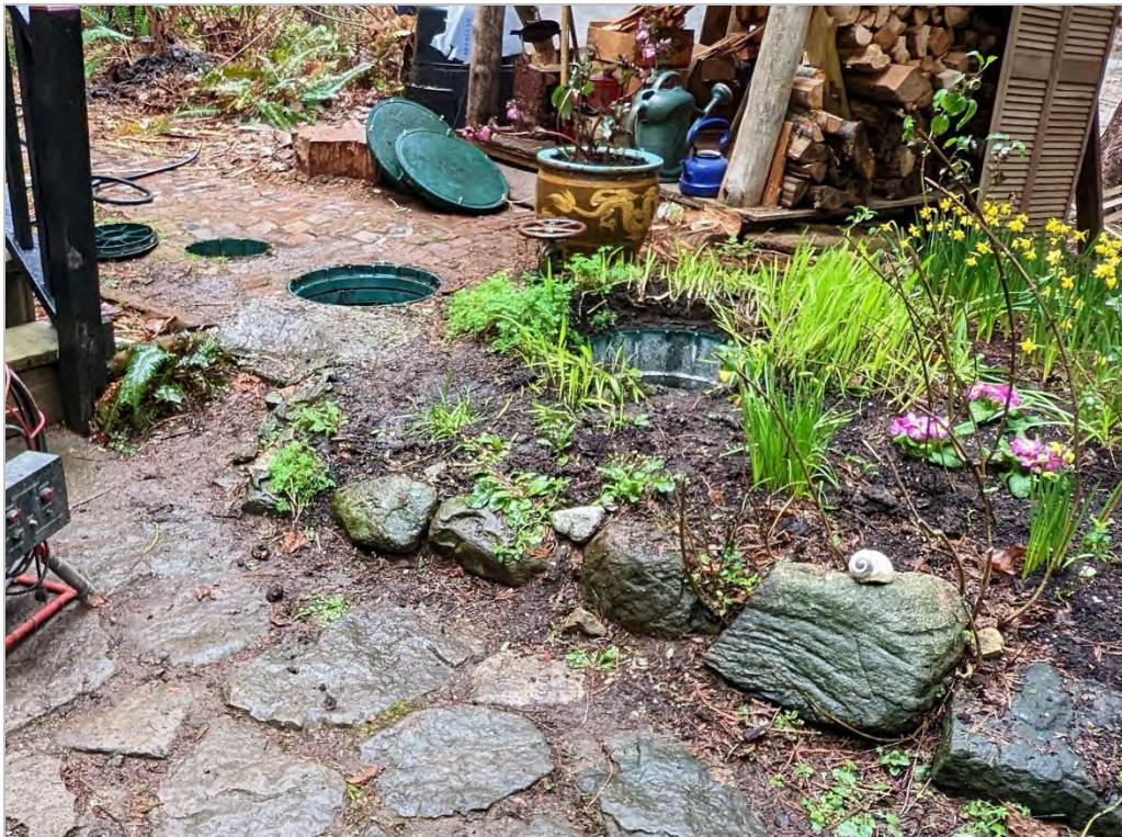
Picture 1: Septic tank location
