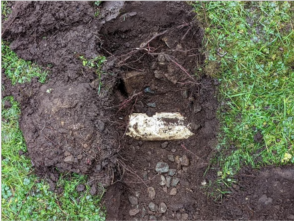
Picture 8: Exposed section of the septic field
