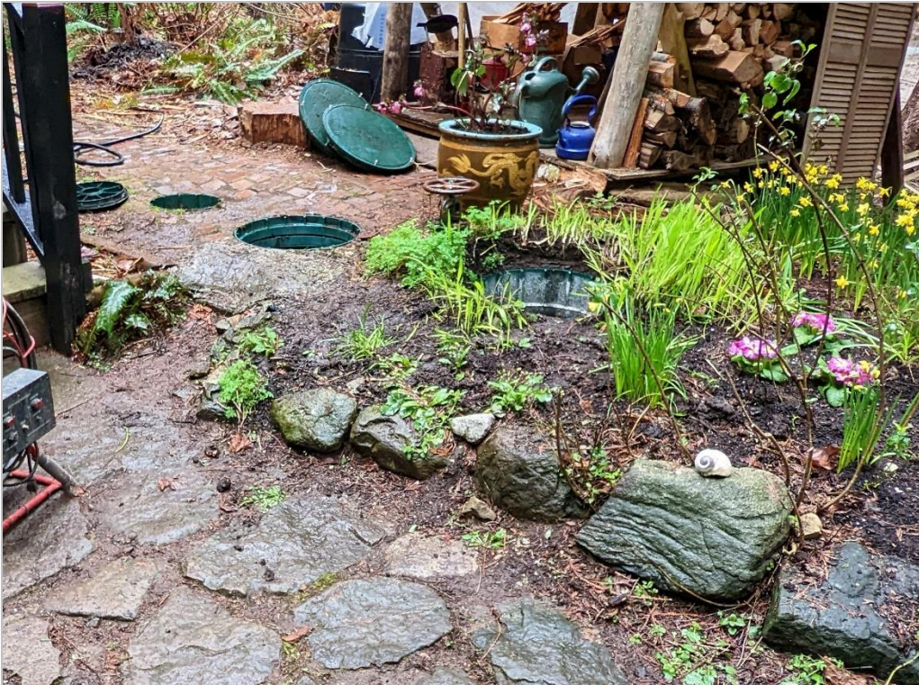
Picture 1: Septic tank location
