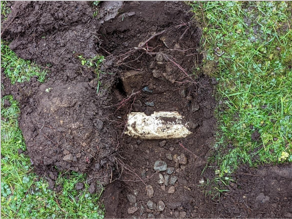
Picture 8: Exposed section of the septic field
