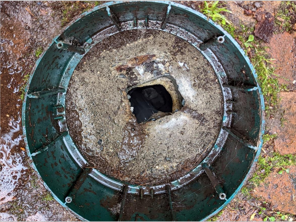
Picture 3: Inlet maintenance hatch
