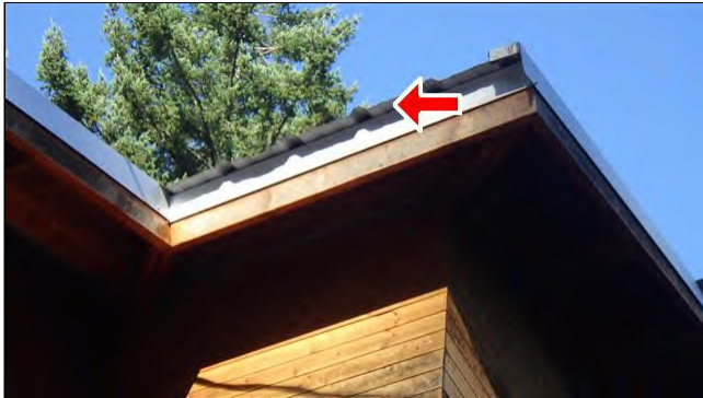
1.9 RAIN GUTTERS / EAVETROUGHES (Picture 1)
