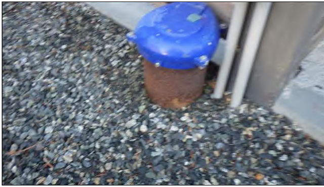
12.0 WATER PIPING (Picture 3)
