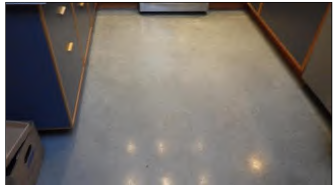
8.1 FLOOR (SLAB) (Picture 8)
