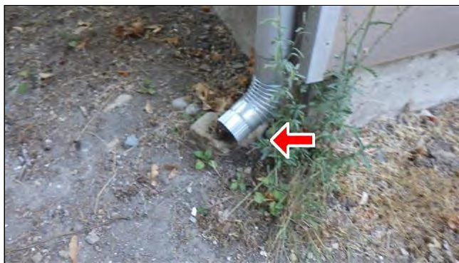
1.10 DOWNSPOUTS / ROOF DRAINS (Picture 3)
