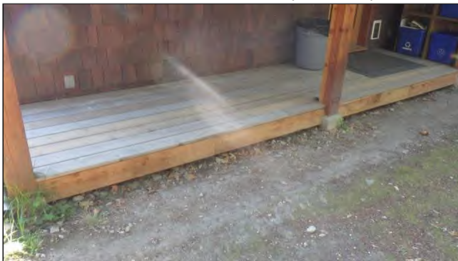
2.4 PORCH(ES) / DECK(S)#1 (Picture 1)
