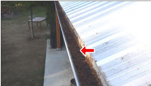
1.9 RAIN GUTTERS / EAVETROUGHES (Picture 3)
