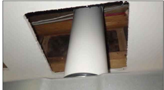
13.1 VENT CONNECTOR (Picture 1)
