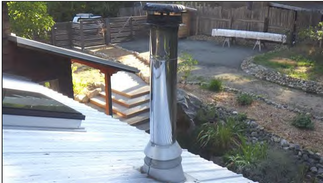
1.3 CHIMNEYS / VENTS (Picture 1)
