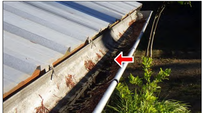
1.9 RAIN GUTTERS / EAVETROUGHES (Picture 4)
