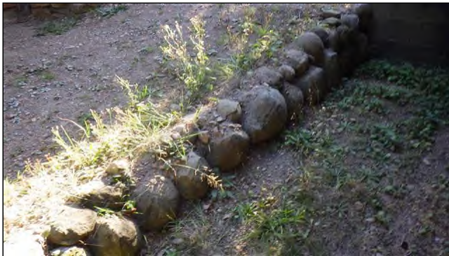
3.5 RETAINING WALL(S) (Picture 1)
