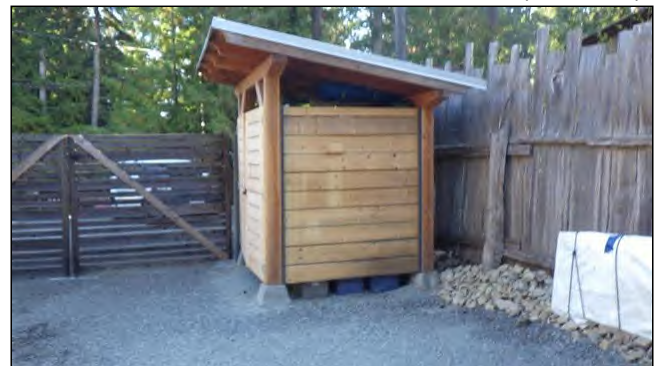
3.6 OUTBUILDINGS, FENCES & SHEDS (Picture 3)
