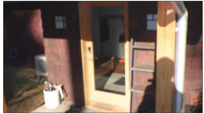
2.1 ENTRY DOORS (Picture 1)
