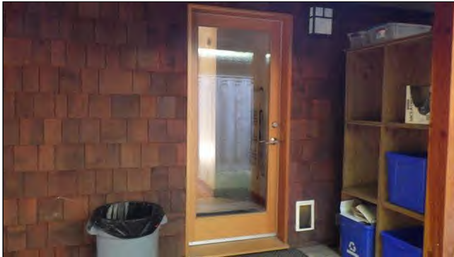
2.1 ENTRY DOORS (Picture 2)
