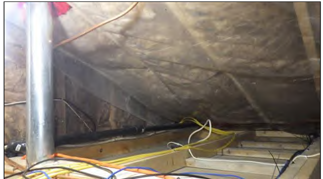
4.0 ROOF FRAMING (Picture 8)
