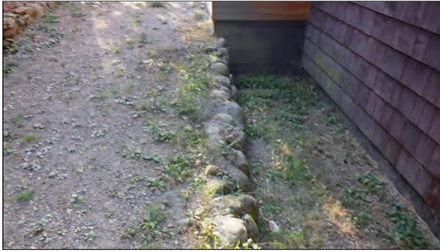
3.3 GROUND SLOPE AT FOUNDATION (Picture 1)
