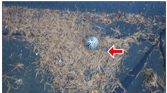
1.10 DOWNSPOUTS / ROOF DRAINS (Picture 2)
