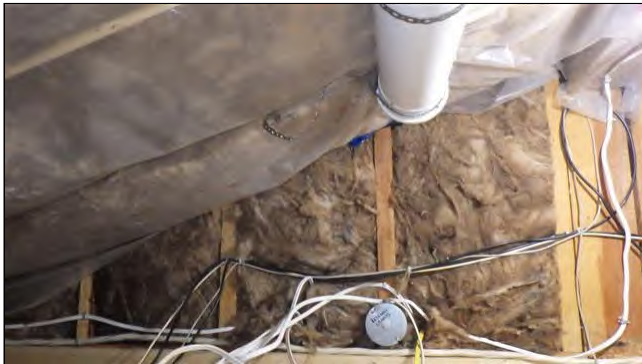
4.0 ROOF FRAMING (Picture 7)
