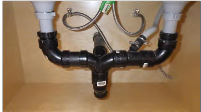
12.2 DRAIN / WASTE PIPING (Picture 1)
