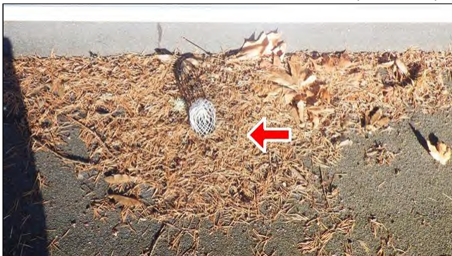
1.10 DOWNSPOUTS / ROOF DRAINS (Picture 1)
