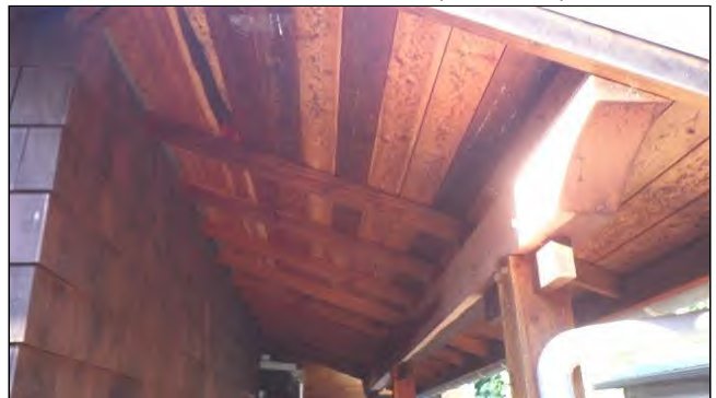
4.0 ROOF FRAMING (Picture 10)
