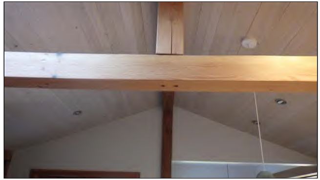
4.0 ROOF FRAMING (Picture 4)
