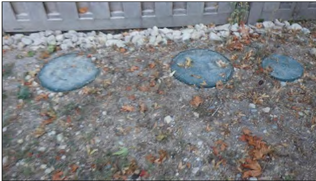
12.2 DRAIN / WASTE PIPING (Picture 2)
