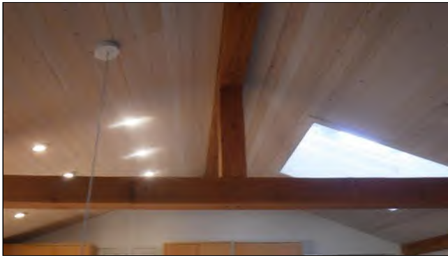
4.0 ROOF FRAMING (Picture 3)
