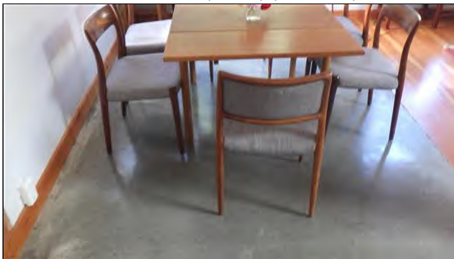
8.1 FLOOR (SLAB) (Picture 9)
