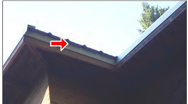
1.9 RAIN GUTTERS / EAVETROUGHES (Picture 2)
