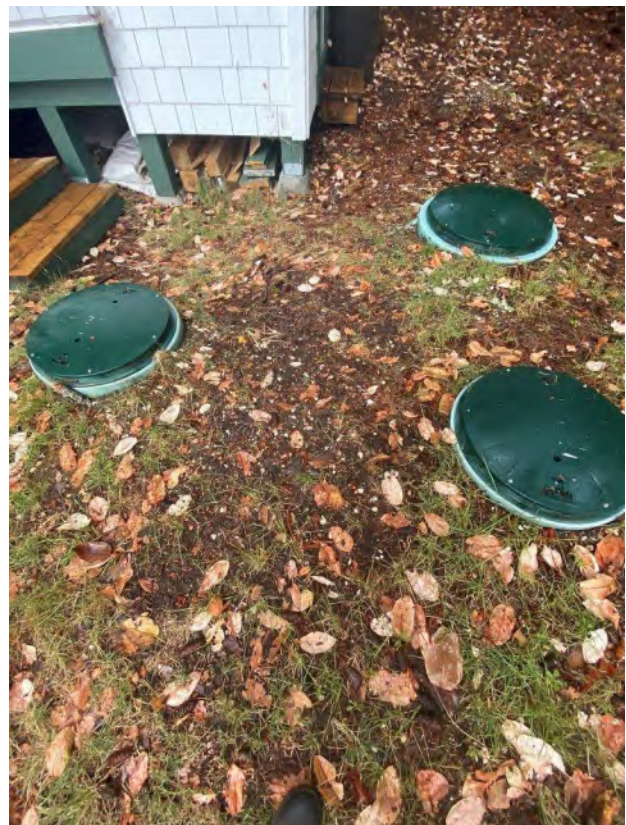
2.9 Septic tanks and pump chamber
