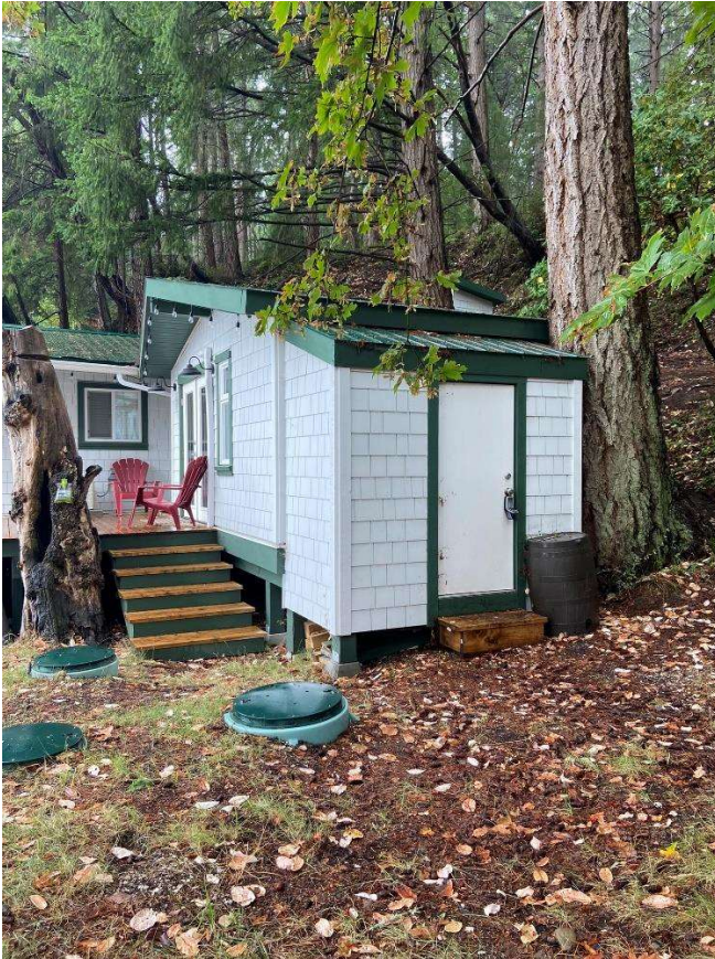
2.10 Eastern portion of cottage and septic tanks
