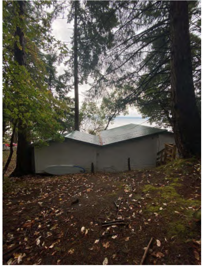
2.11 Back of cottage facing south
