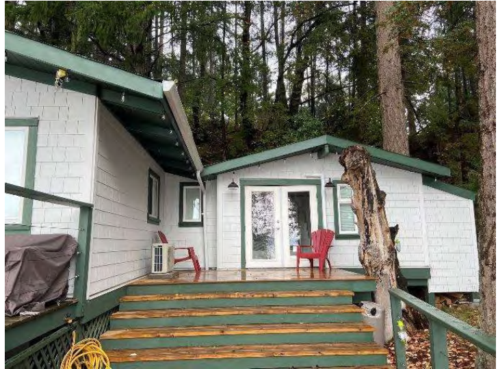
2.13 Eastern portion of cottage and deck
