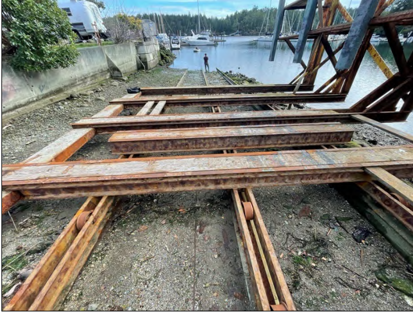
Photo 1. The shipway from the upper intertidal, looking east.
