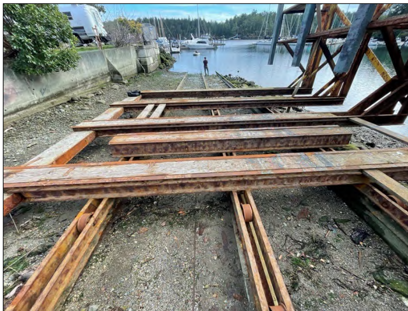
Photo 1. The shipway from the upper intertidal, looking east.
