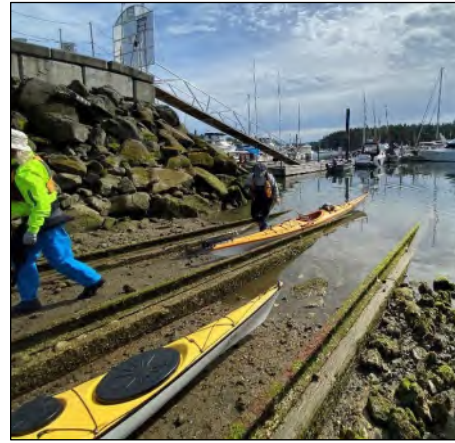
(B) Existing rip rap in front of the lock block wall. Photo is facing north from the intertidal area.
