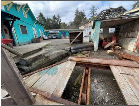
Photo 4. (A) Backshore area with shipway infrastructure. Photo is facing west onshore from the upper intertidal area.
