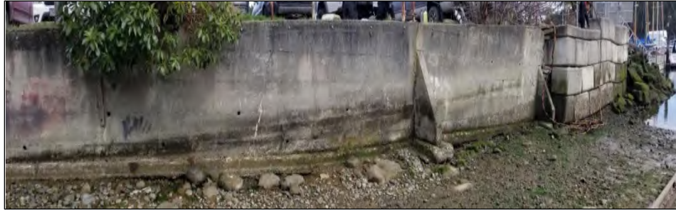
Photo 3. Existing cast-in-place and lock block concrete retaining wall on the north side of the shipway.
