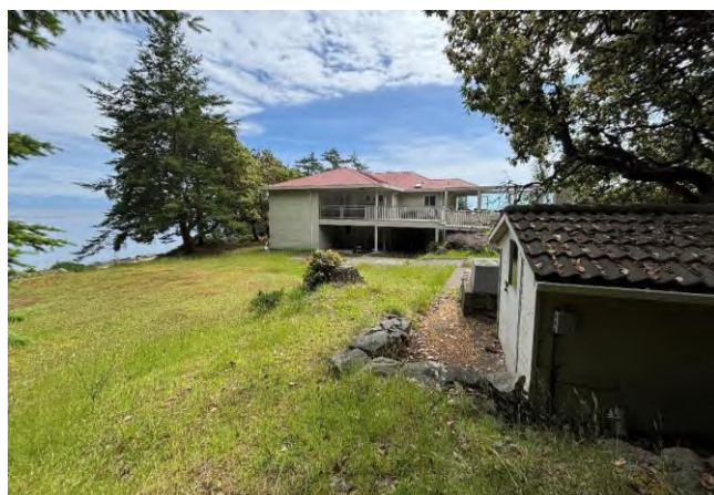
Photo 5: View of the pumphouse and electrical box sheds.
