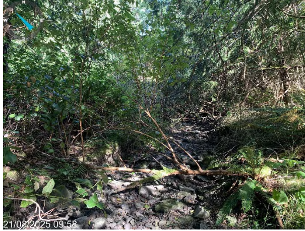
Photo 13: View of Dick Brook upstream of the Pond. Dry channel conditions and bank scouring observed (21/08/2025).
