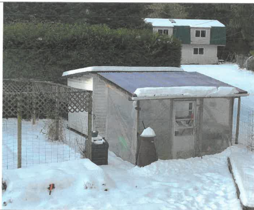
Structure #2 Storage Shed
