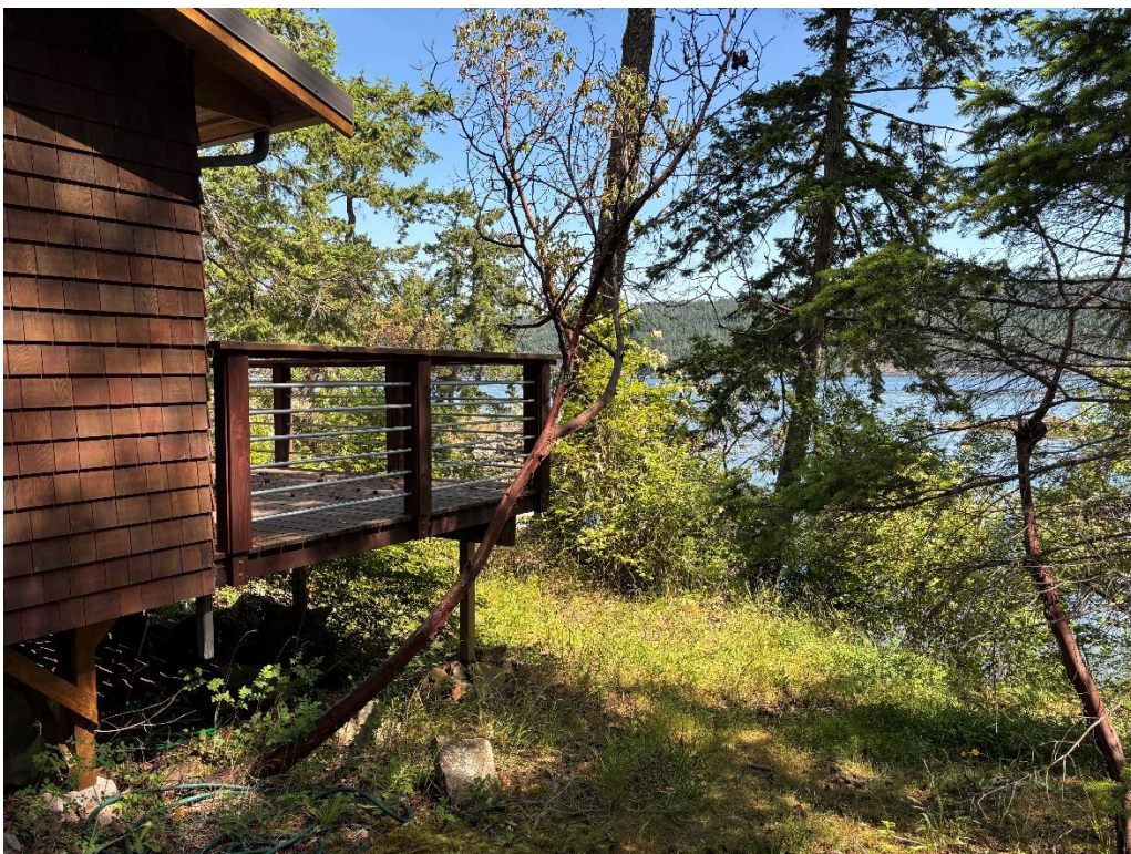
Figure 2.2.2 E Existing house and deck, and undeveloped road (Looking north-east)
