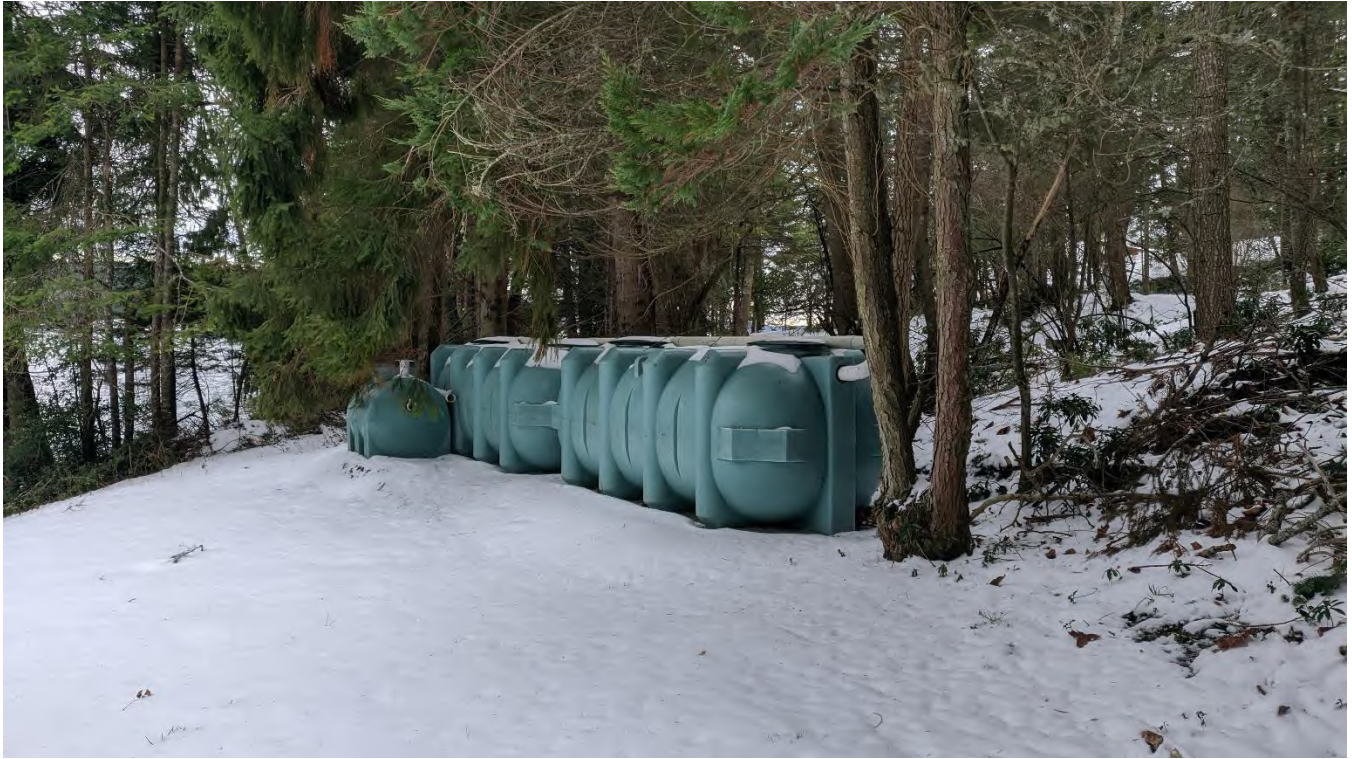
Figure 2.3.1 Septic Tanks (Looking South-East)
