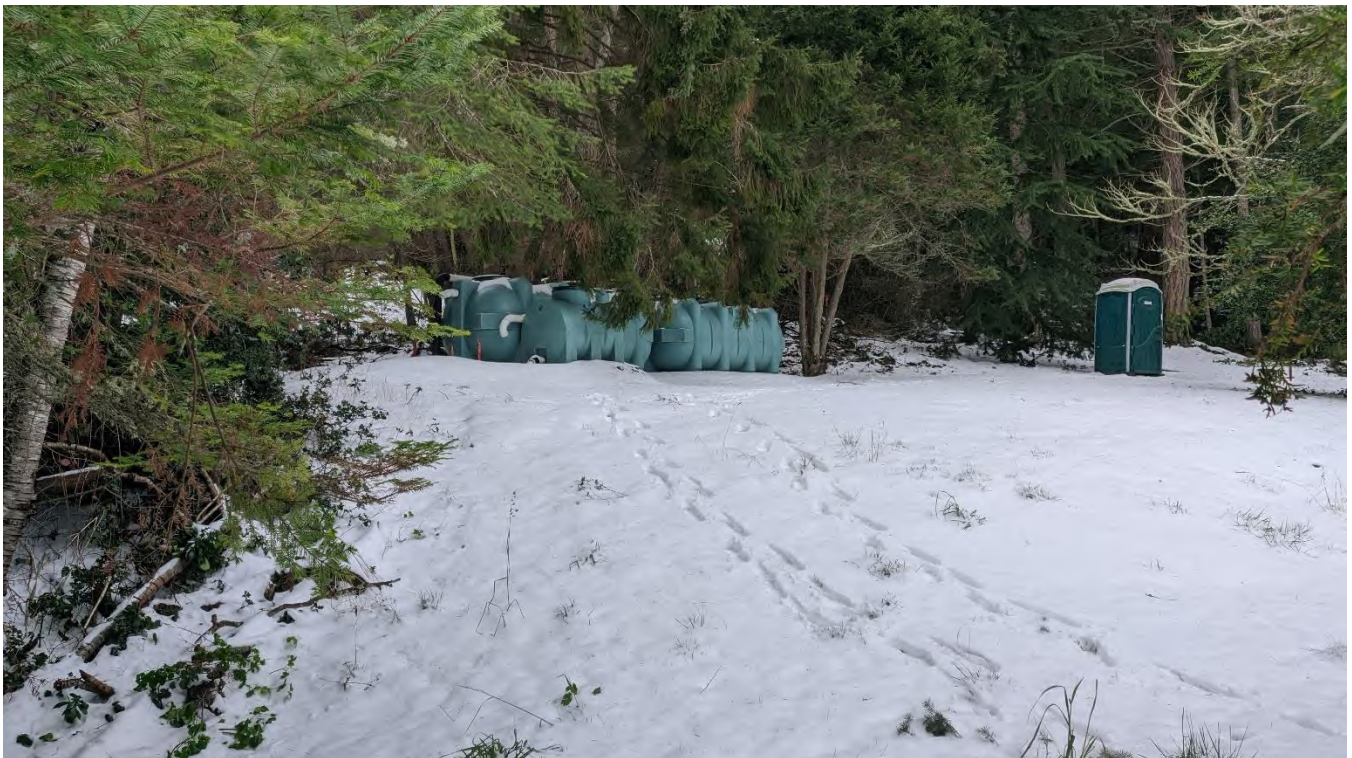
Figure 2.3.4 Septic Tanks and DPA boundary marker (Looking West)
