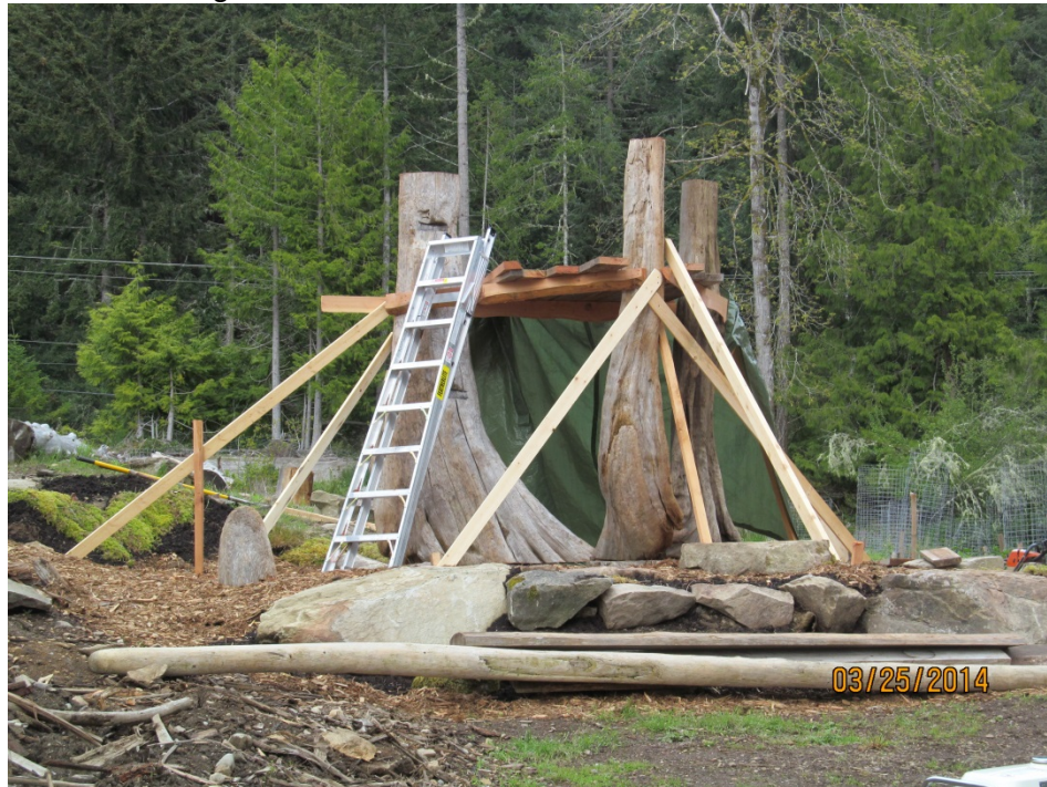
Figure 15: Information Kiosk under Construction
