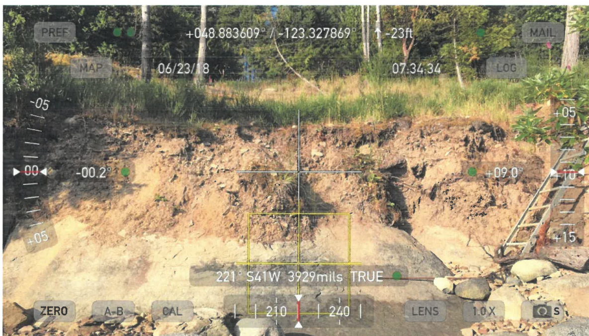
Photo 4. Bedrock outcrop located along shoreline of subject property, downgradient of proposed treatment and dispersal field, facing SW.
