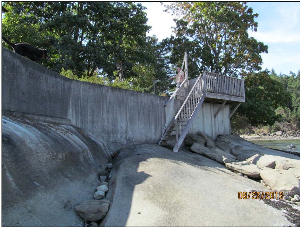
Picture 2: Retaining wall and stairs included in requested variance
