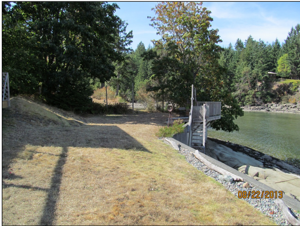
Picture 4: Rear yard looking west (retaining wall along the right)
