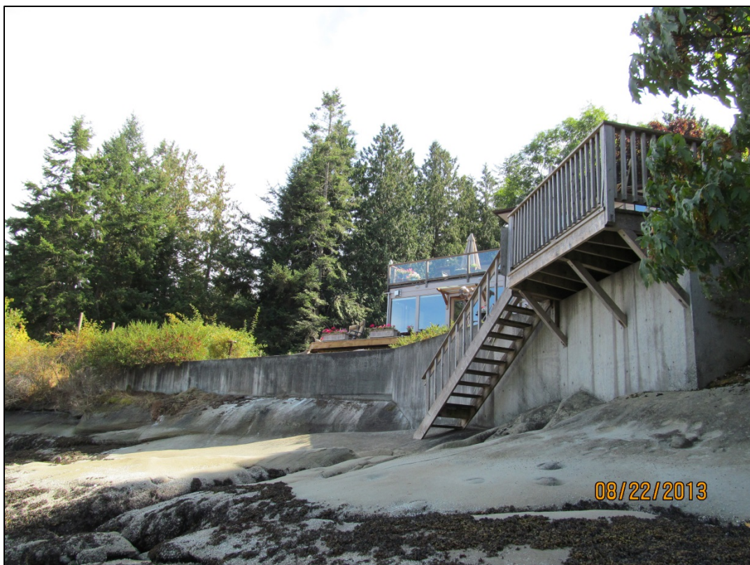
Picture 1: View of retaining wall from foreshore
