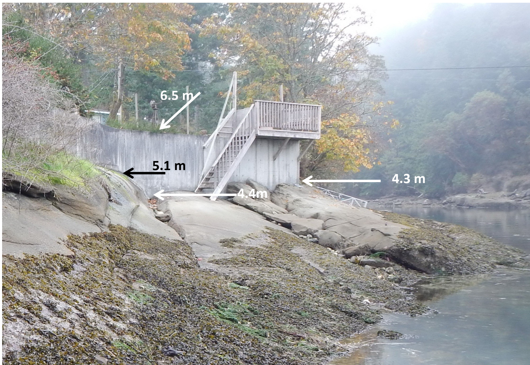
Figure 4. Measured elevations along the seawall. Elevations are referenced to tidal datum.
