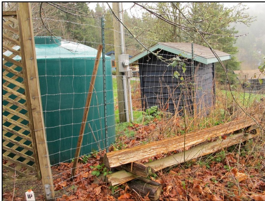
Figure 6: Encroaching cistern and electrical shed (East view)
