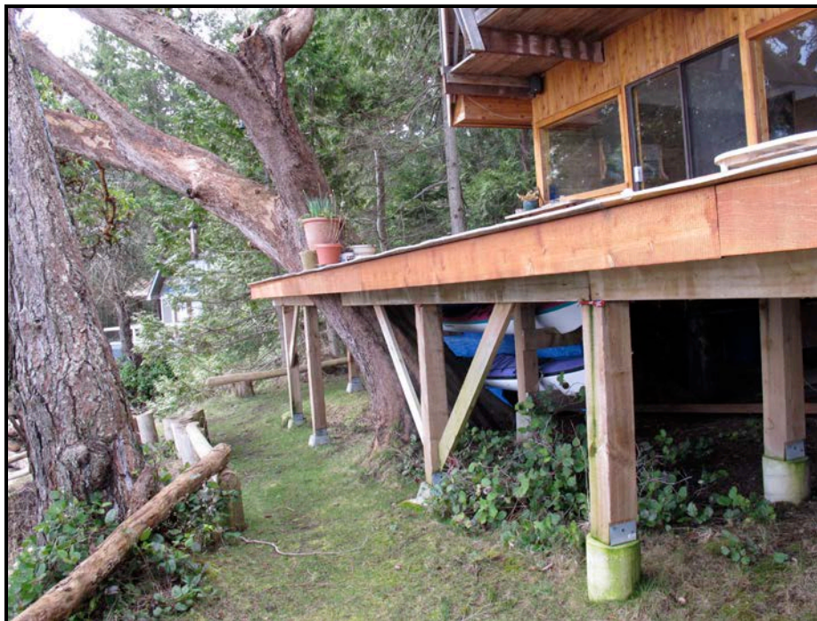
Figure 9: Reconstructed deck facing the sea (east side)
