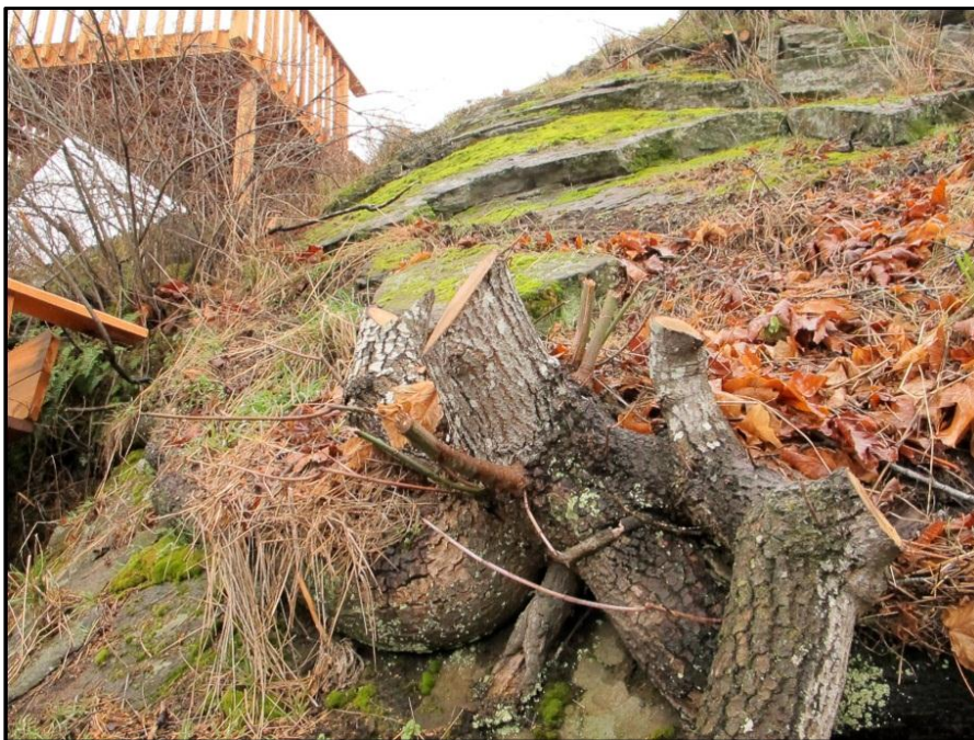
Figure 12: Tree cutting in proximity to stair construction
