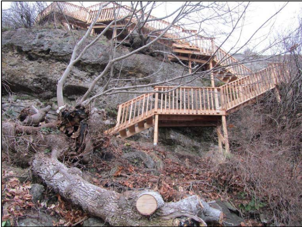
Figure 11: Extent of stairs looking up from the beach
