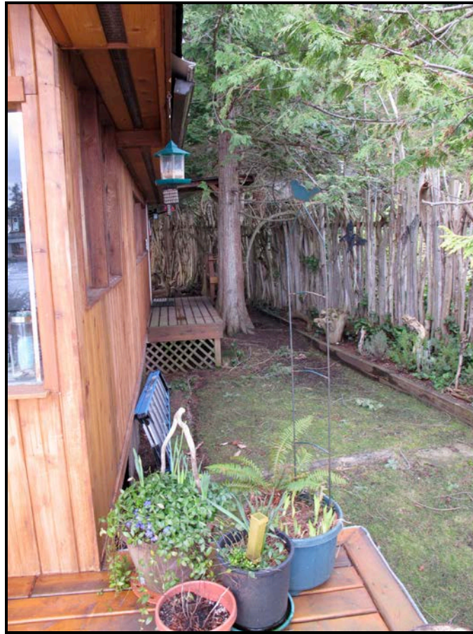
Figure 11: North side of residence
