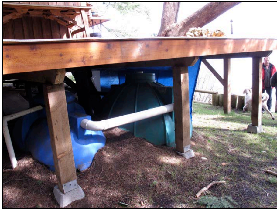
Figure 8: Deck over septic tanks (south side)
